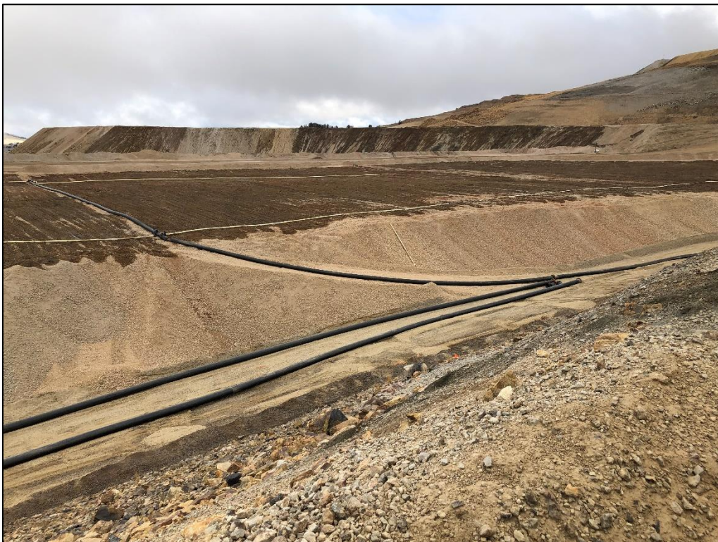
Photo 2. View looking northwest from top of HGM platform, showing SGVLF leaching surface. No solution ponding greater than 3 feet x 3 feet in size was observed.
