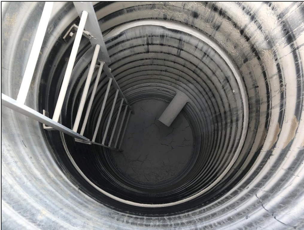
Photo 16. View looking inside LDS sump AG-LDS-12, showing sump dry during inspection.
