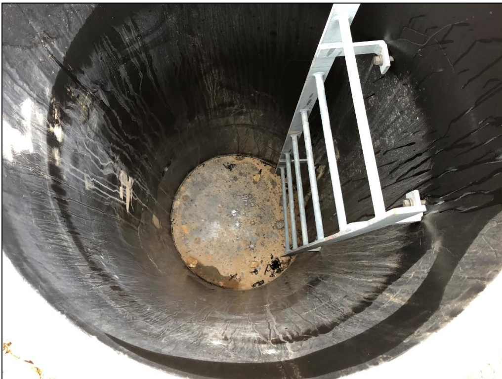
Photo 6. View looking inside LDS sump SG-LDS-1, showing sump dry during inspection.
