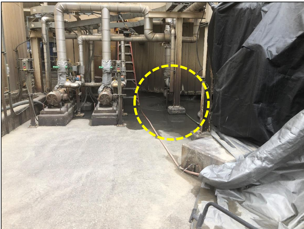
Photo 20. View looking across secondary containment for high pH thickener, located on east side of HGM. High pH thickener tank was being drained during the inspection for cleaning (drainage area circled).
