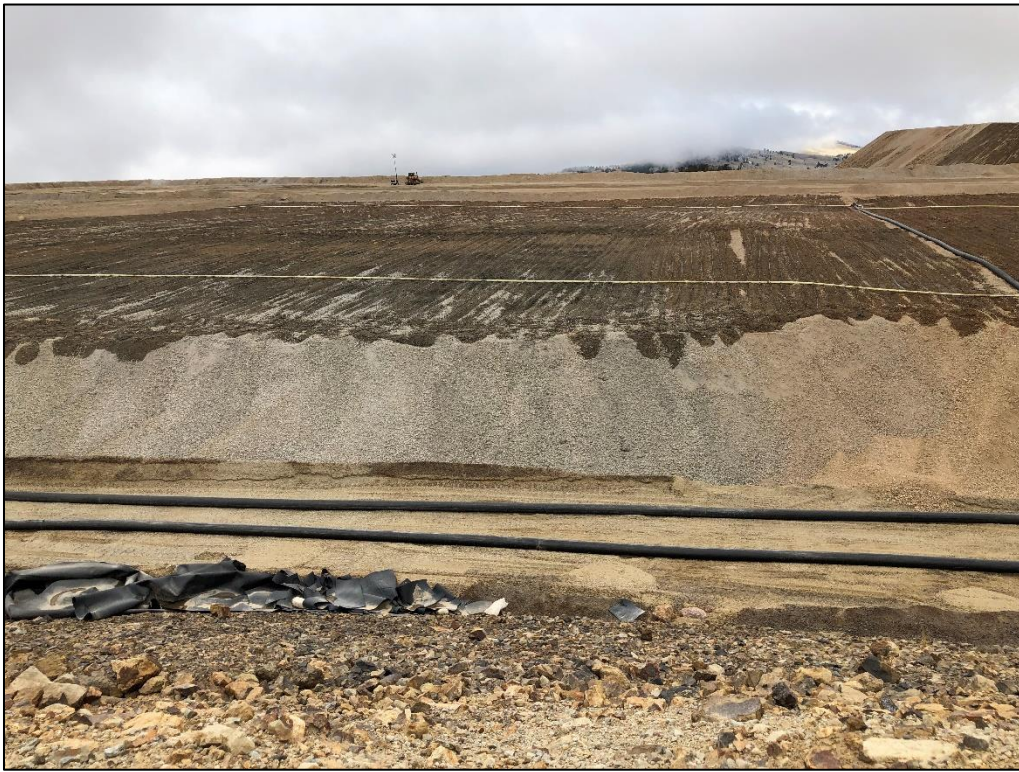
Photo 1. View looking west from top of HGM platform, showing SGVLF leaching surface. No solution ponding greater than 3 feet x 3 feet in size was observed.
