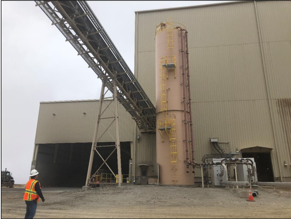
Photo 25. View looking west showing 330 ton silo located at southeastern edge of HGM proposed for relocation to SGOSA in TR-114.
