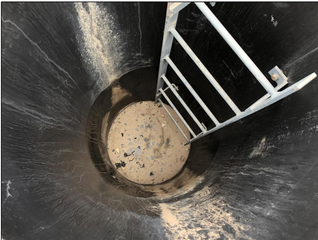
Photo 10. View looking inside LDS sump SG-LDS-3, showing sump dry during inspection.
