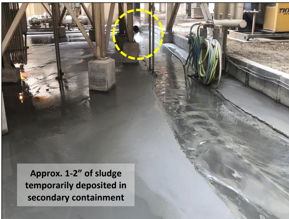
Photo 22. View looking across western half of secondary containment for processed ore thickener, located on east side of HGM. Water from high pH thickener sump was being discharged (circled) into this structure during inspection.
