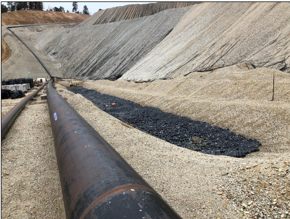
Photo 4. View looking northwest across sump at SGVLF toe filled with bird balls. This sump appeared to be dry during the inspection.
