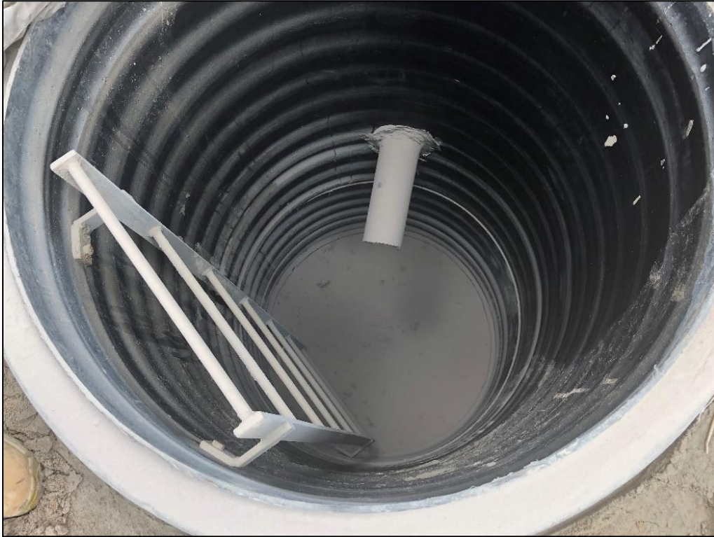
Photo 17. View looking inside LDS sump AG-LDS-13, showing sump dry during inspection.
