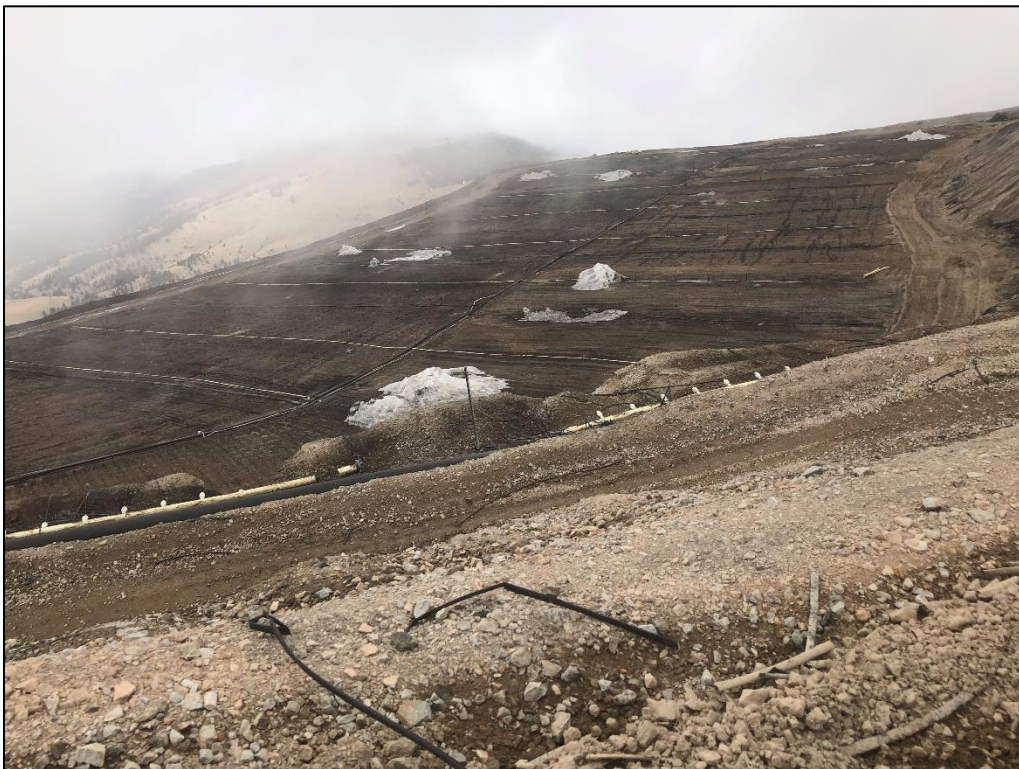
Photo 12. View looking across leaching surface of AGVLF at the 10,400 foot elevation. No solution ponding greater than 3 feet x 3 feet in size was observed. Note ice present on leaching surface.
