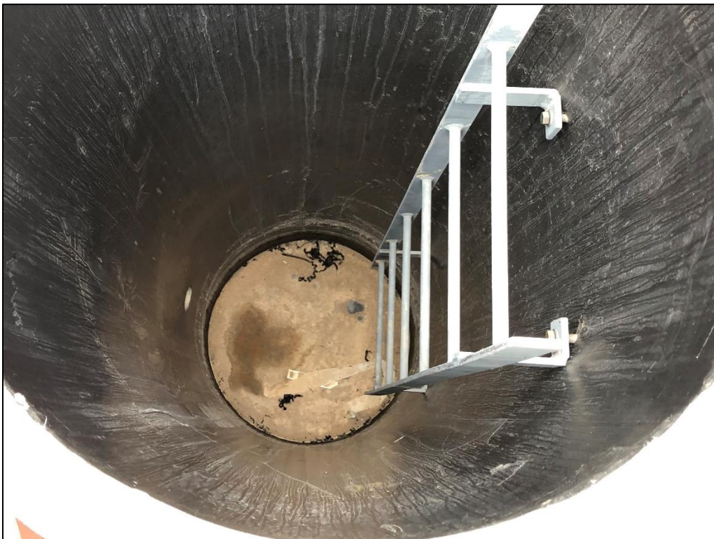
Photo 8. View looking inside LDS sump SG-LDS-2, showing sump dry during inspection.
