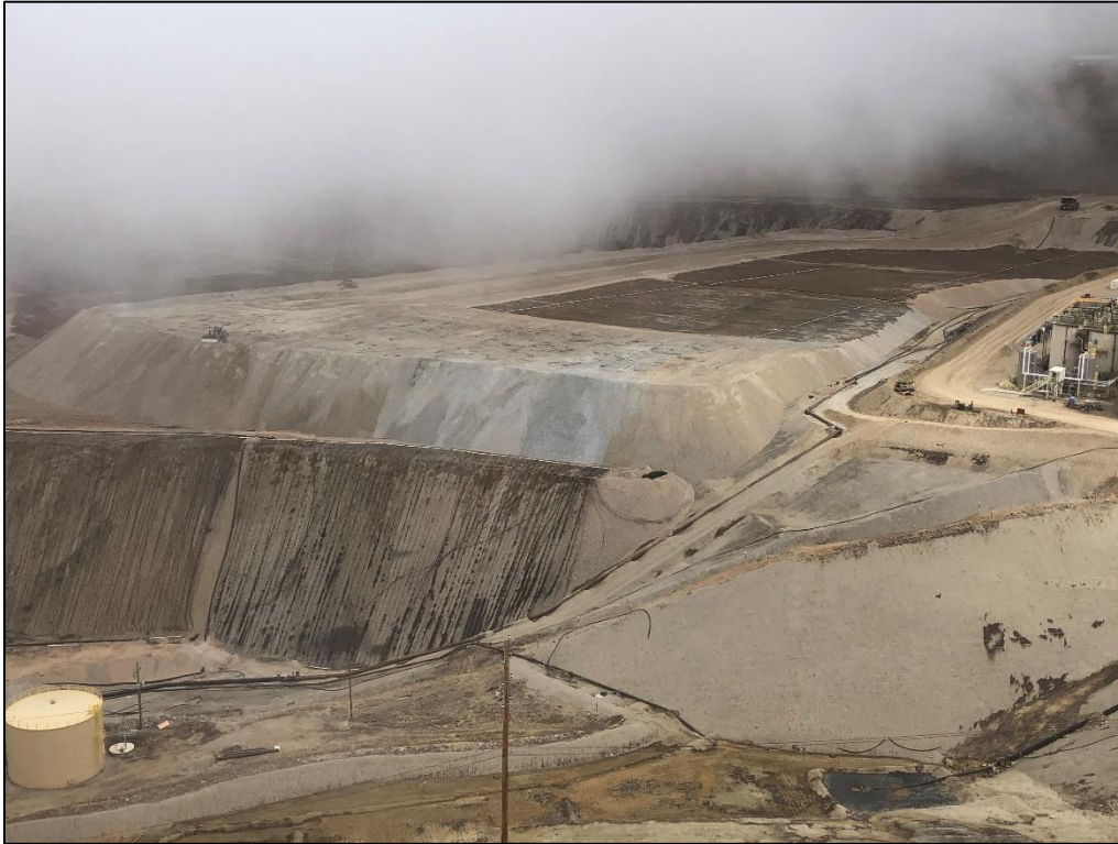
Photo 3. View looking northwest from overlook located south of HGM, showing SGVLF leaching surfaces. No solution ponding greater than 3 feet x 3 feet in size was observed. Note dense fog reducing visibility of northwestern portion of SGVLF.
