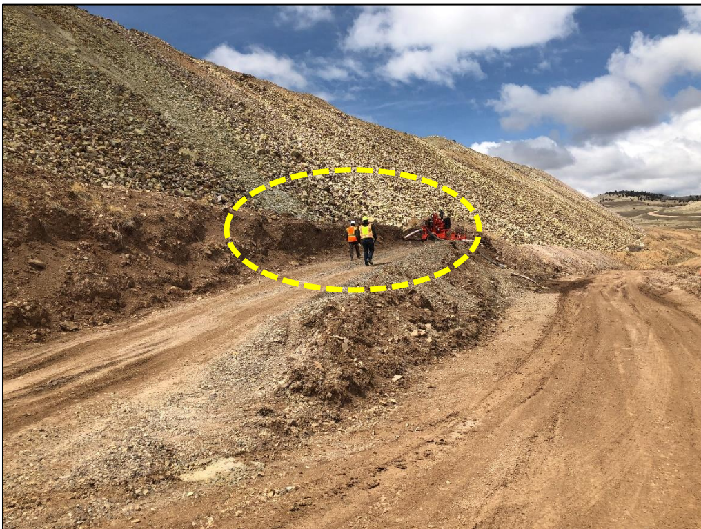
Photo 28. View looking northwest, showing location of seep accumulation trench at eastern toe of ECOSA (circled).
