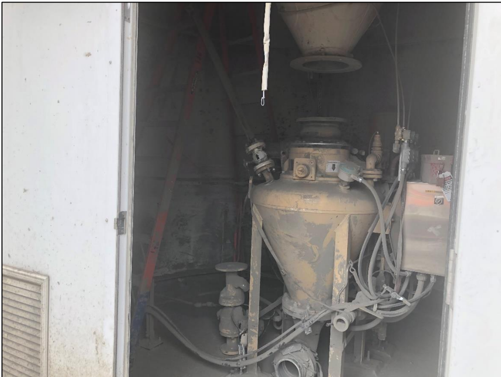
Photo 26. View looking inside 330 ton silo located at southeastern edge of HGM proposed for relocation to SGOSA in TR-114.
