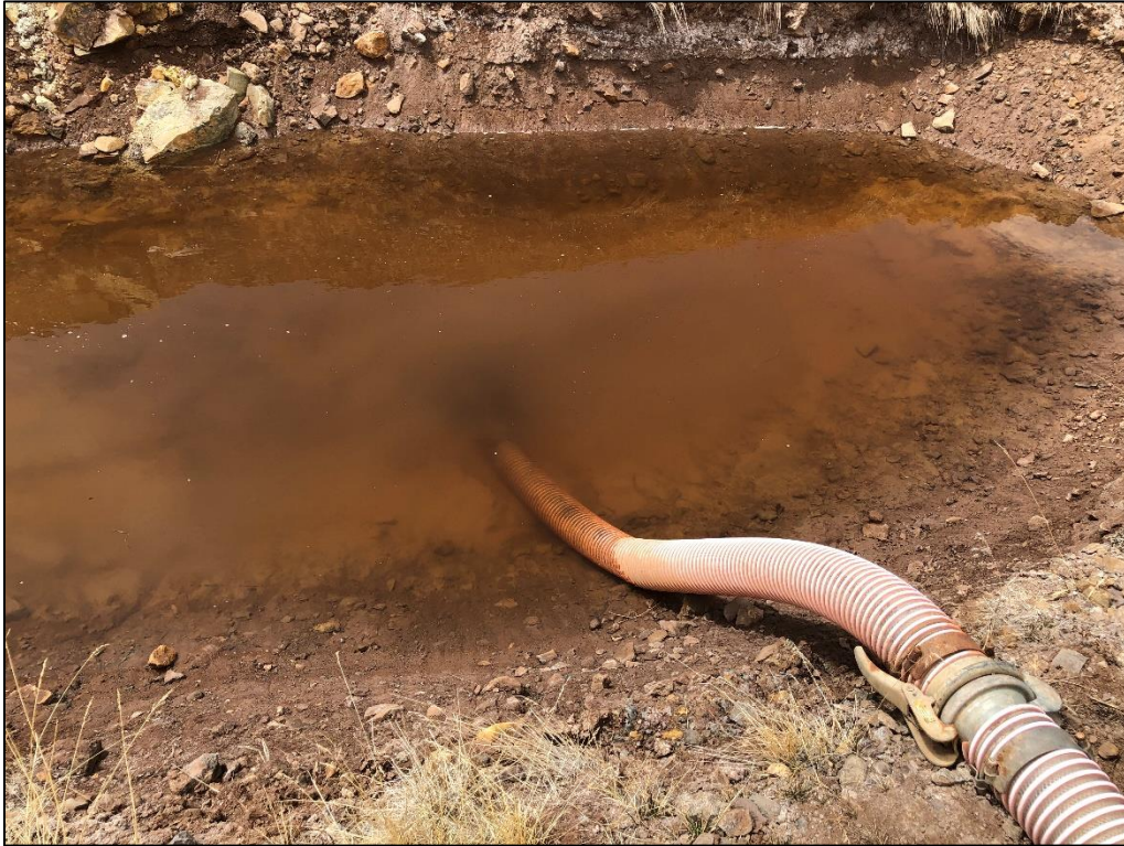
Photo 29. View of seep accumulation trench at eastern toe of ECOSA, showing approximately 2-1/2 feet of water present in trench during inspection.
