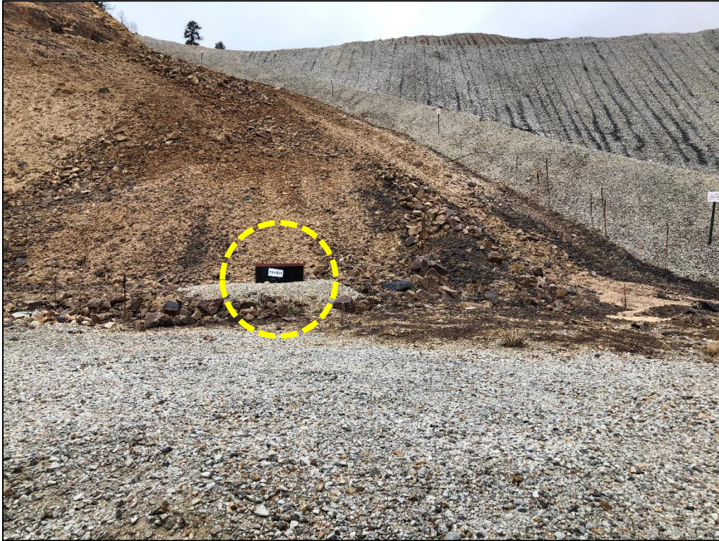
Photo 7. View looking north, showing location of LDS sump SG-LDS-2 (circled) at southwestern edge of SGVLF.
