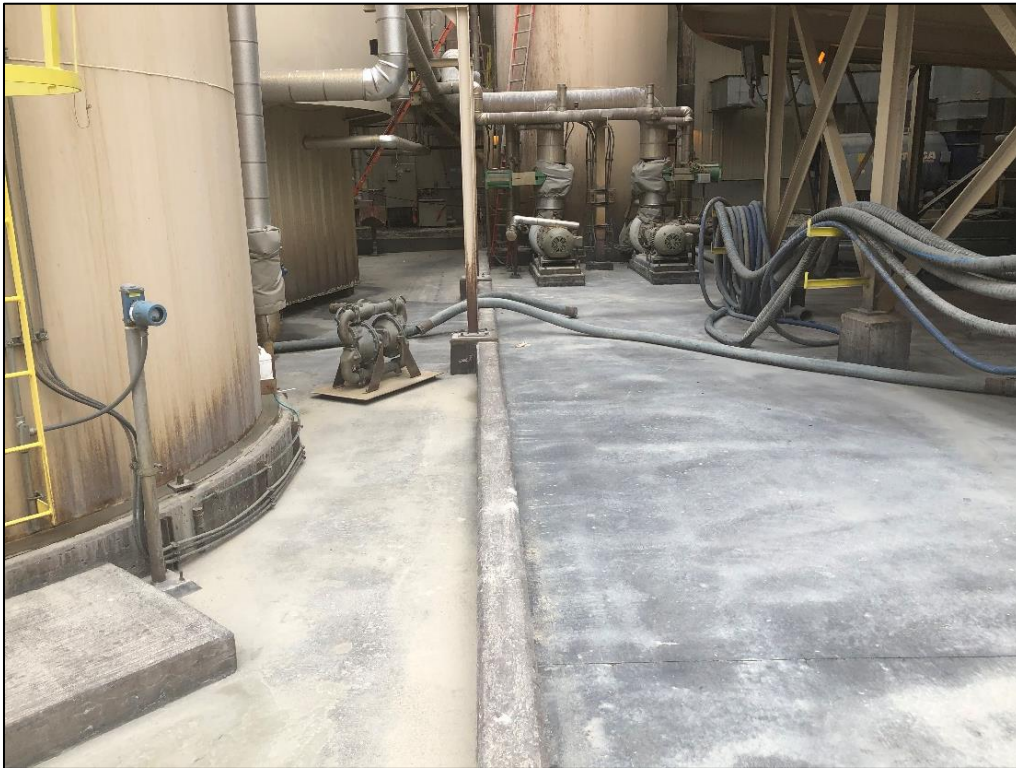
Photo 21. View looking across secondary containment for high pH thickener (left) and processed ore thickener (right), located on east side of HGM. Water was being pumped from high pH thickener sump to secondary containment of processed ore thickener during inspection (note hose at center).
