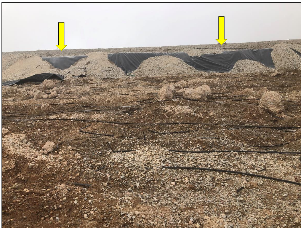
Photo 14. View looking west across top of AGVLF, showing Phase III area (indicated) proposed for use in a leach cell study (in TR-113). Approximately 3 feet of previously processed crushed ore has already been placed on a geomembrane liner in this area.
