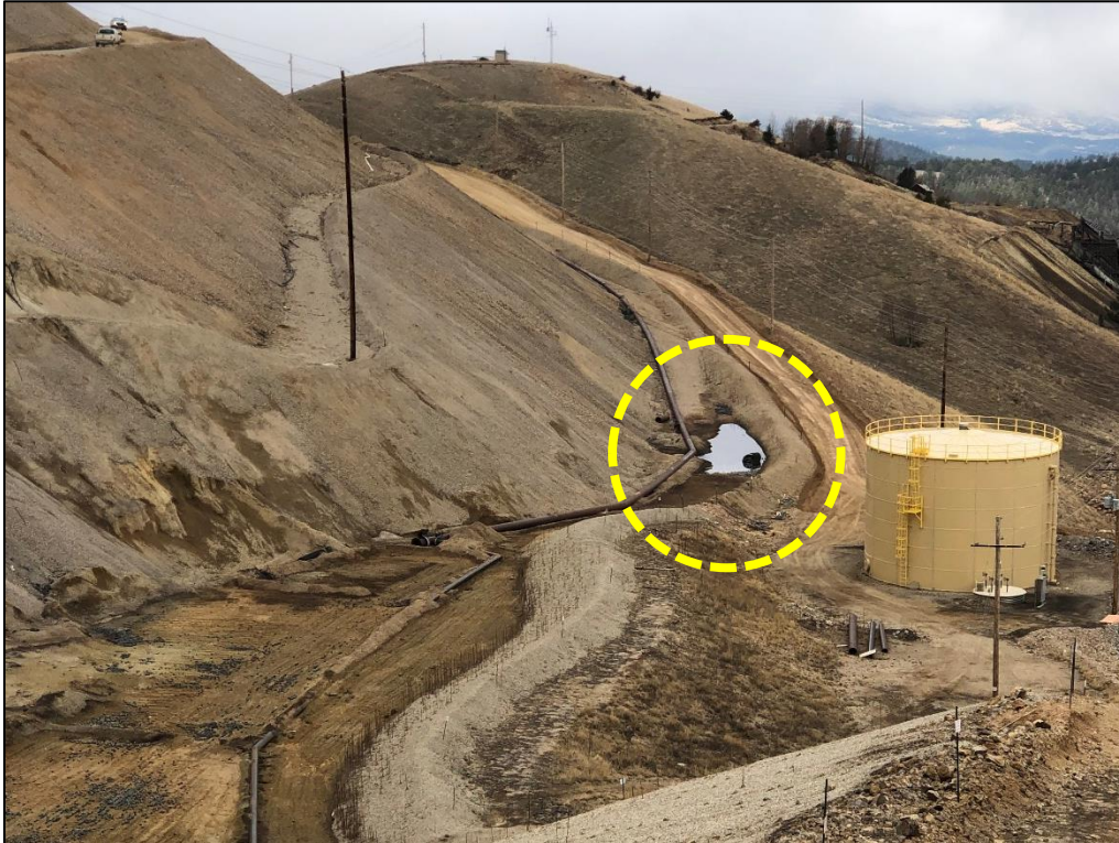
Photo 13. View looking southwest from top of HGM platform, showing ponding inside toe berm of AGVLF (circled) which the operator indicated is meteoric water.
