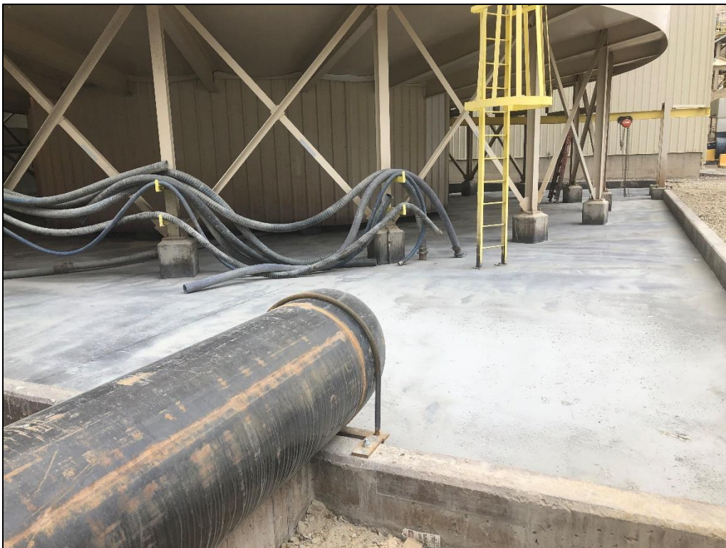
Photo 24. View looking across eastern half of secondary containment for processed ore thickener, located on east side of HGM. Note this portion of the structure had no reduction in capacity during the inspection.
