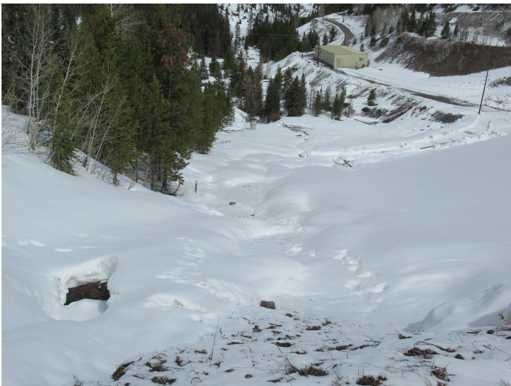
View of sink hole along the left abutment of the East Branch Dam from CR 3
