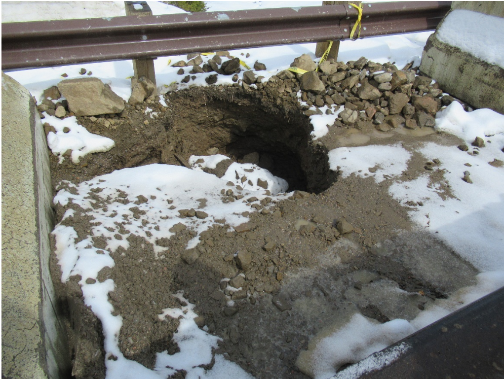
View of sink hole above the East Branch Dam left abutment along CR 3 shoulder
