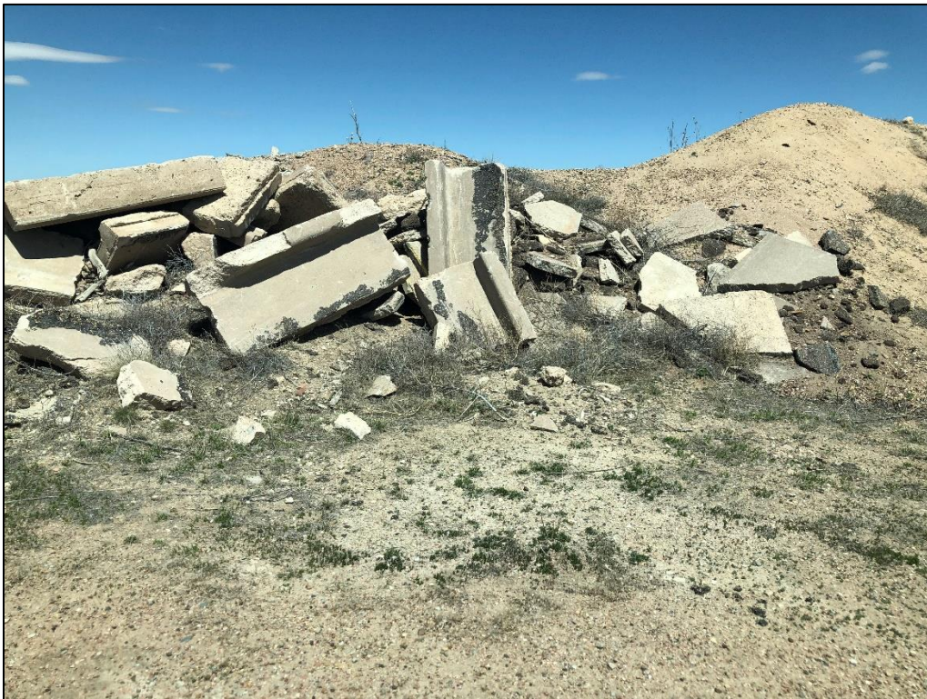
Photo 14. View looking north across eastern parcel showing waste rock and concrete rubble piles stored southwest of ponds which can be used as pond backfill for reclamation.
