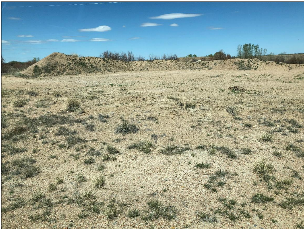
Photo 12. View looking north across eastern parcel showing overburden stockpile stored south of smaller pond which can be used as pond backfill for reclamation.
