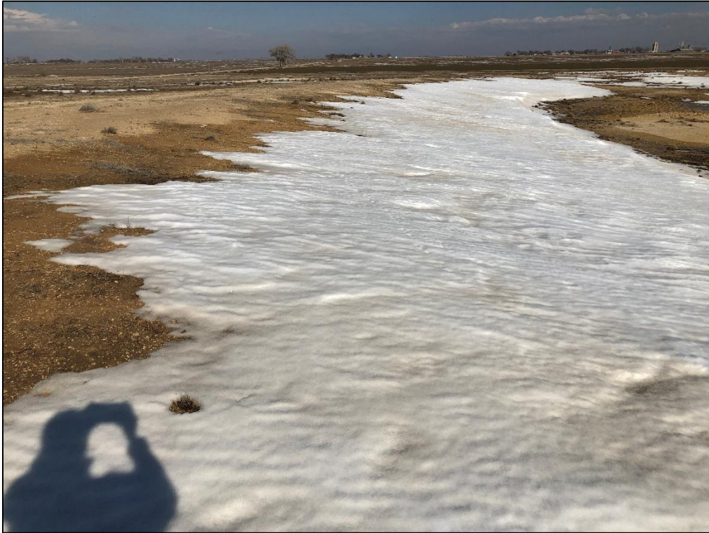
Photo 3. View looking east across northern pit slope, graded flatter than 3H:1V.
