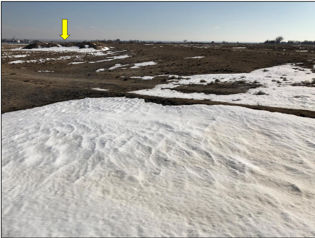
Photo 1. View looking southwest across western pit slope, graded flatter than 3H:1V. Note material stockpile stored on pit floor (indicated with arrow in background).
