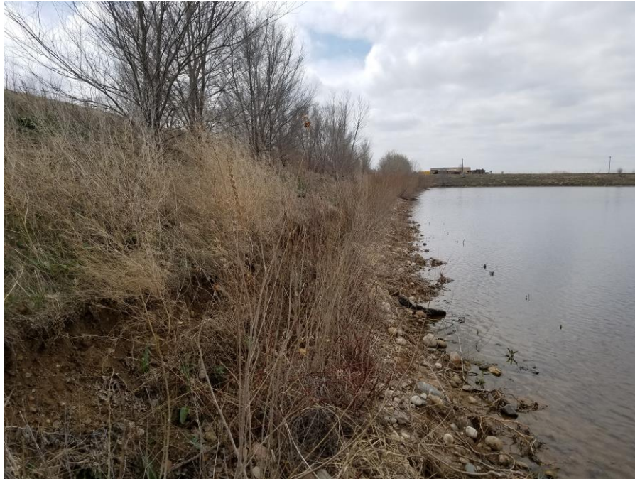
Figure 5. Shore cutting on the southern pit slope of Mining Area I.
