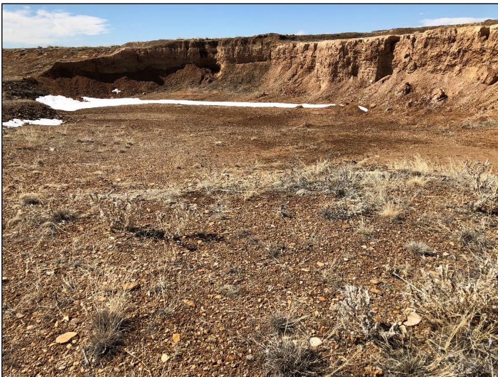
Photo 4. View looking west across excavation area, showing portion of highwall, which is approximately 10 feet in height with near vertical slopes.
