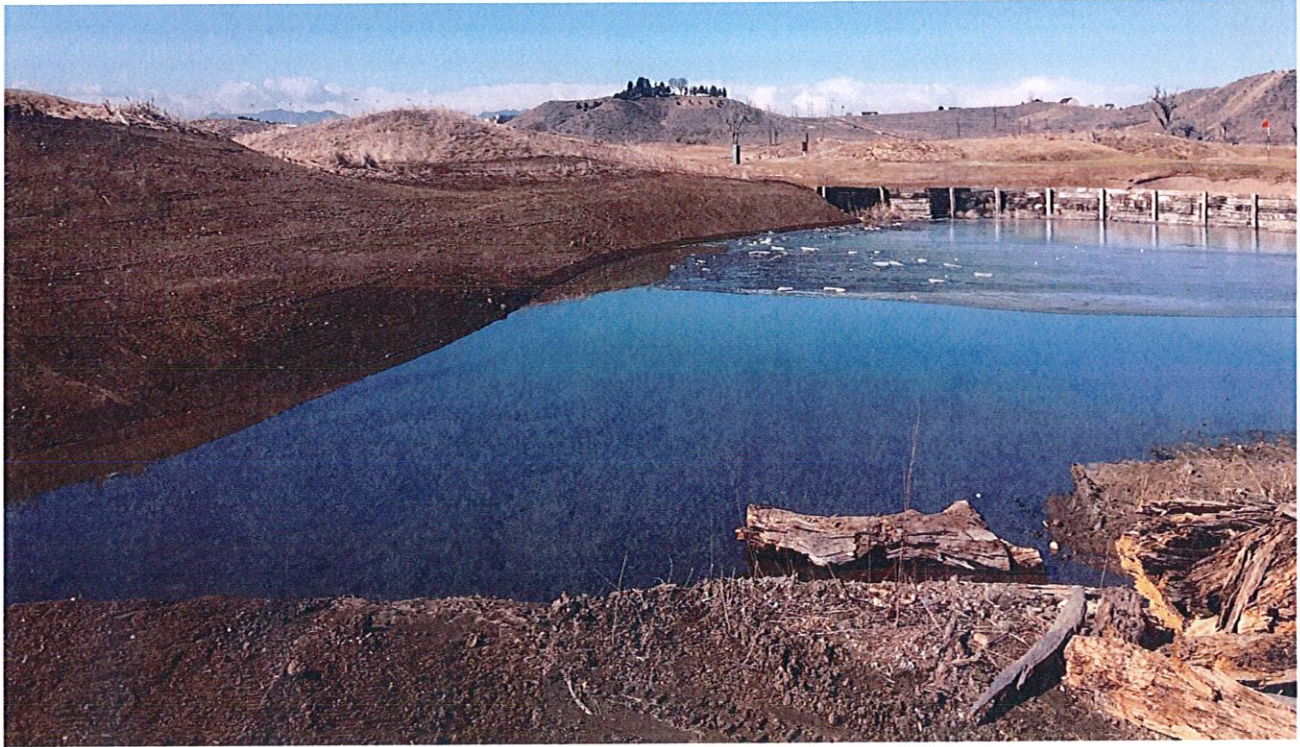
Photo 3 – Photo of final grade of embankment at northernmost area on TR02 Map Area (pre seeding) Note: This area to be seeded and mulch /coconut matting installed as weather/soil conditions allow
