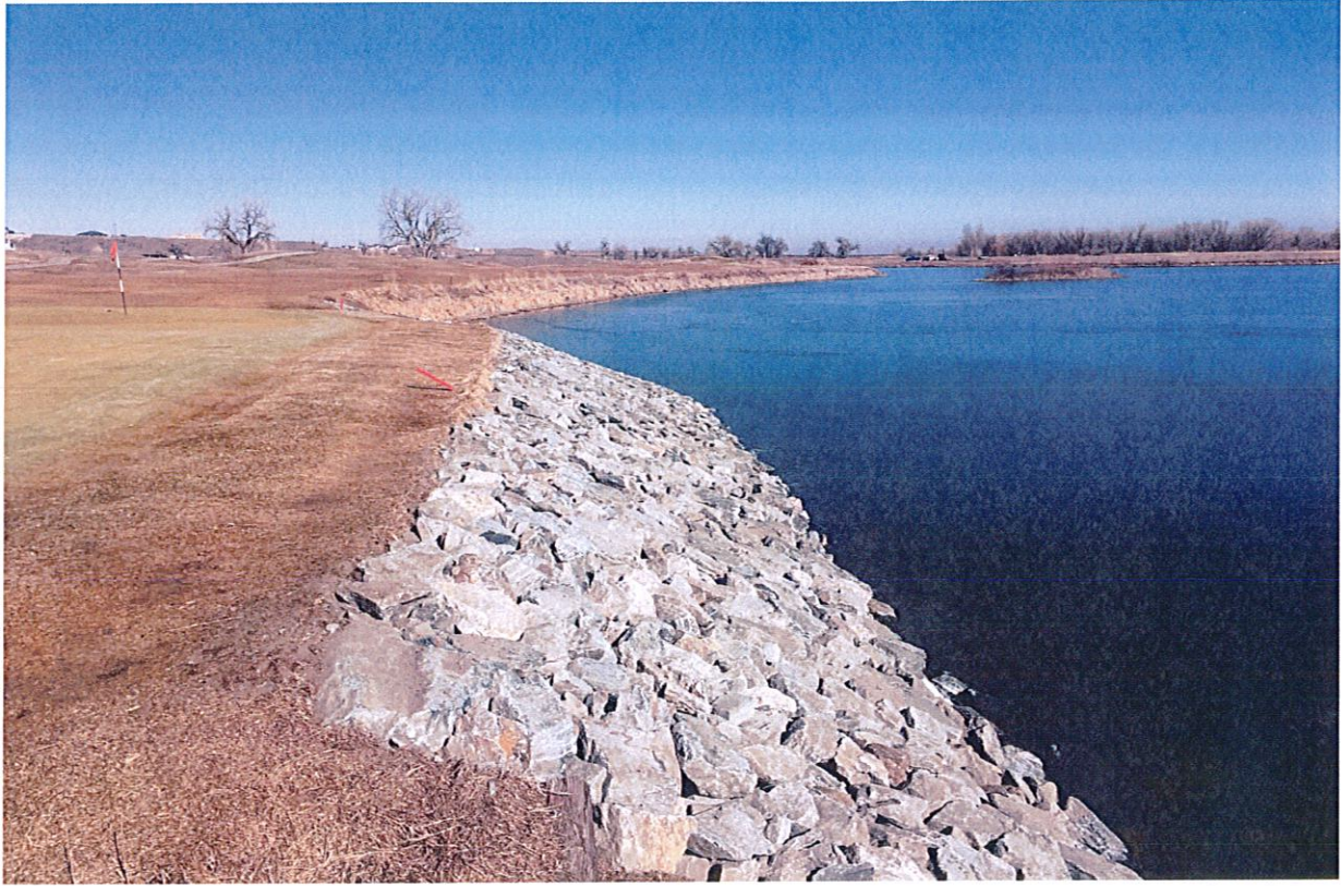
Photo 8 showing western pond bank (Southernmost area on TR02 Map) after rip rap adjacent to green Looking North
