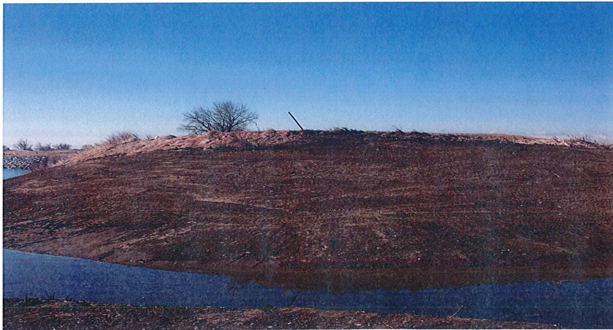
Photo 2 – Photo of final grade of embankment at northernmost area on TR02 Map Area (pre-seeding) Note: This area to be seeded and coconut erosion matting installed as weather/soil conditions allow.
