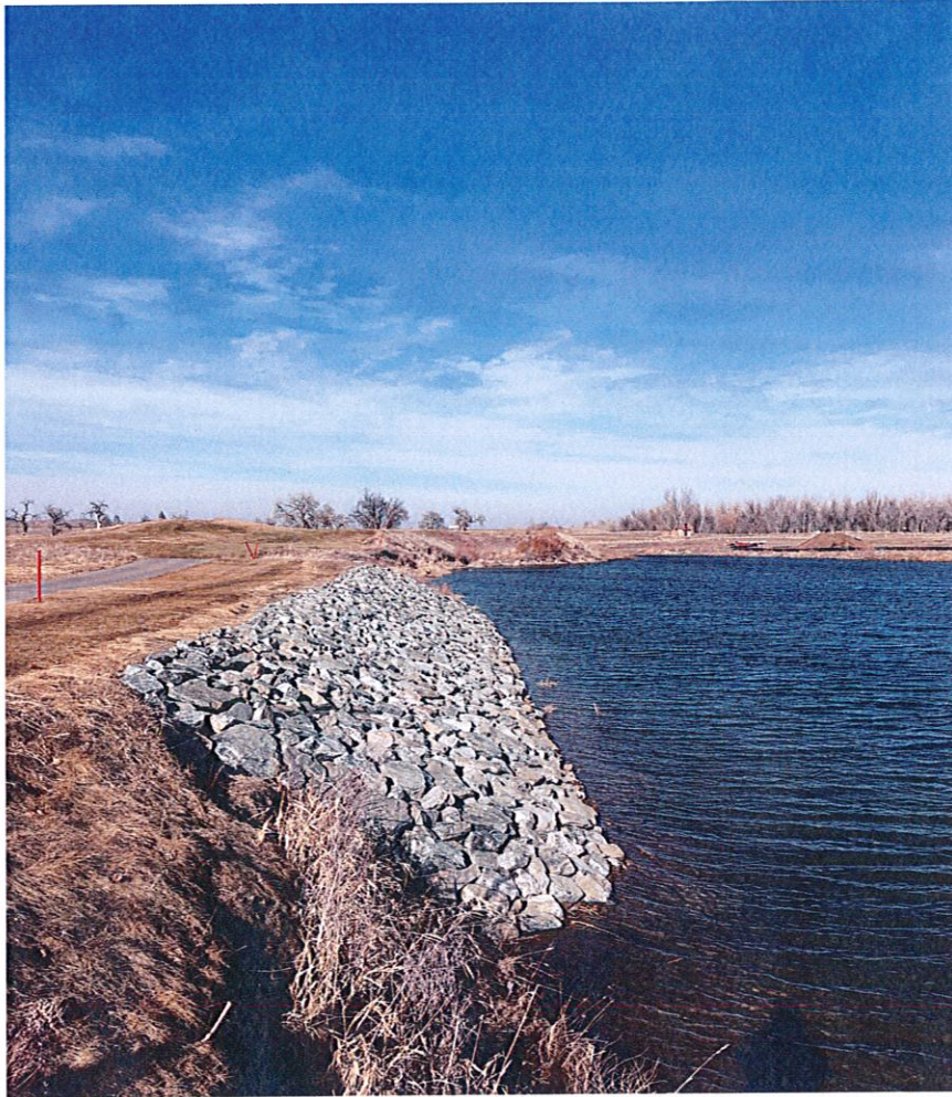
Photo 5 showing western pond bank (central area on TR02 Map) after rip rap installation
