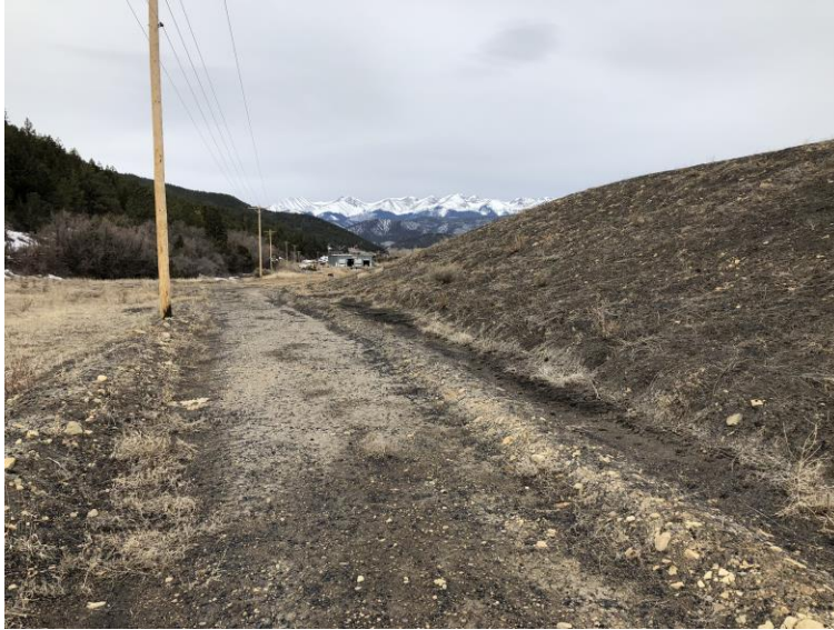
Need for sediment removal from ring ditch around soil pile
