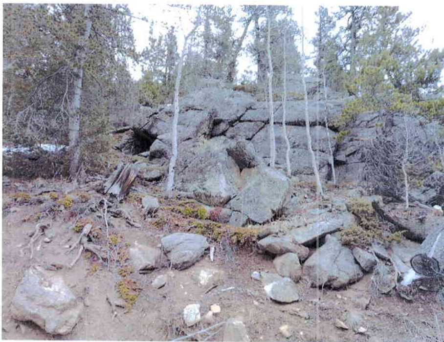
Photo 3 - Rock Slope Above Ute Creek Road (typical)
