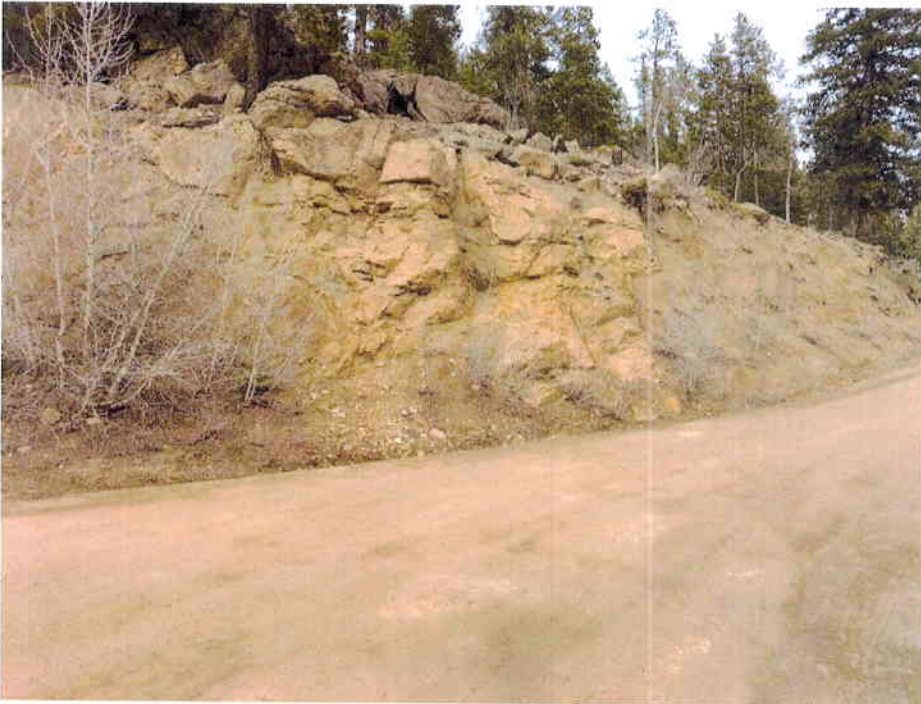
Photo 2 - Ute Creek Road, Road Cut (Typical)
