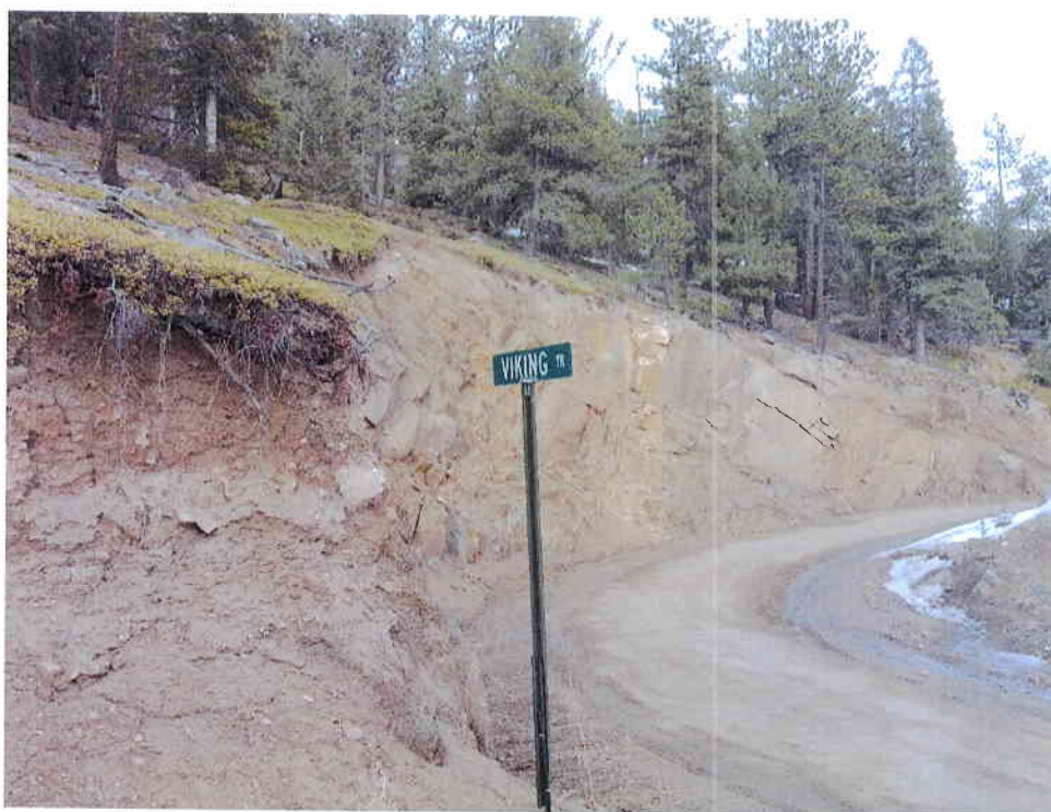
Photo 12 - Rock Cut at Intersection of Ute Creek and Viking Roads
