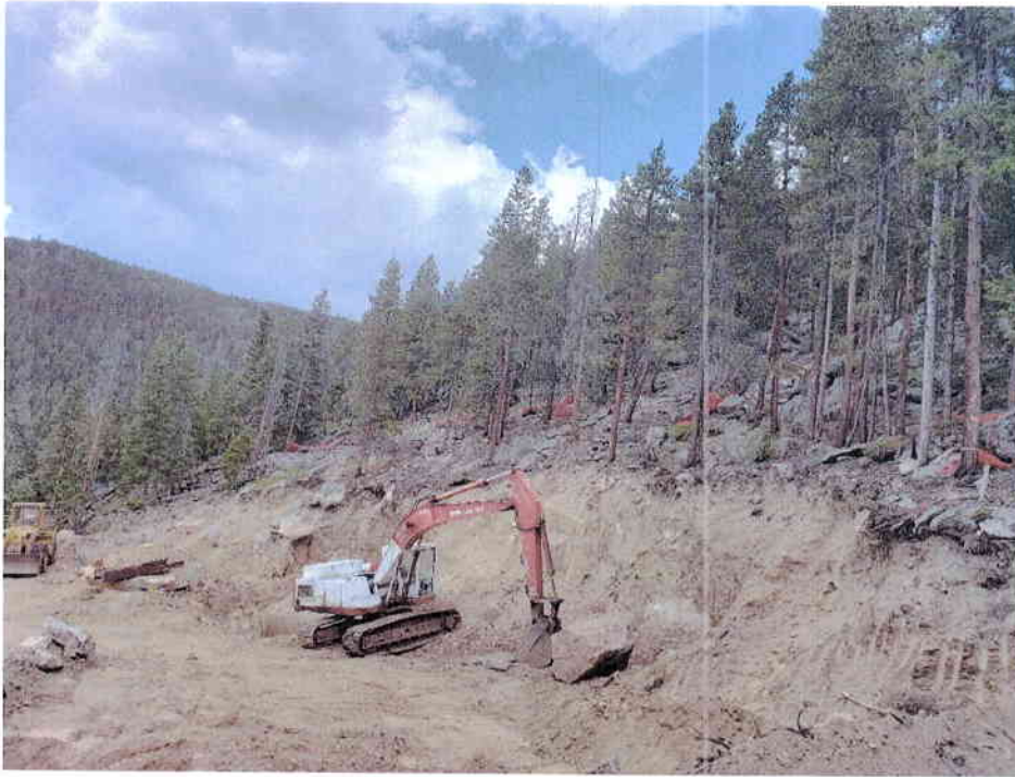
Photo 1 - Working Pad, Trench Area and "Highwall"
