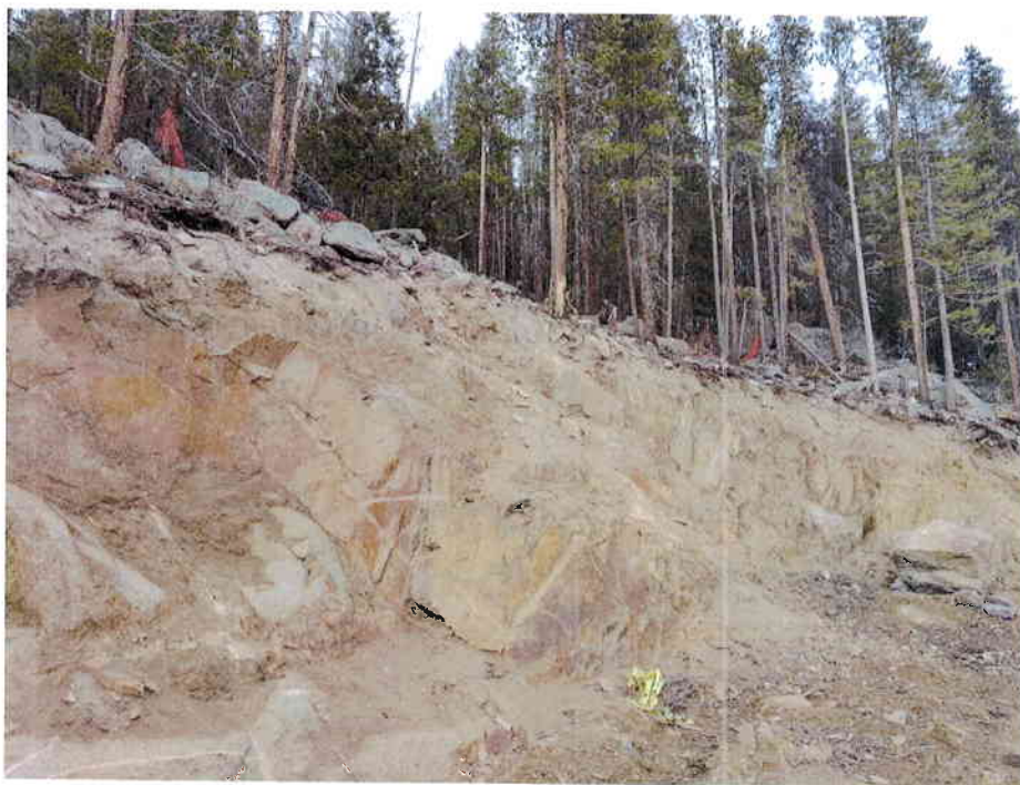
Photo 4 - Mining Area "Highwall"
