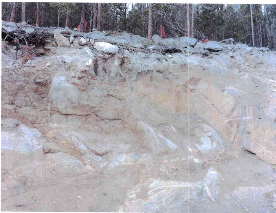
Photo 5 - Mining Area "Highwall"
