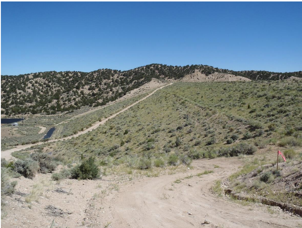
Photo 2. Downstream slope (looking north from left groin).
