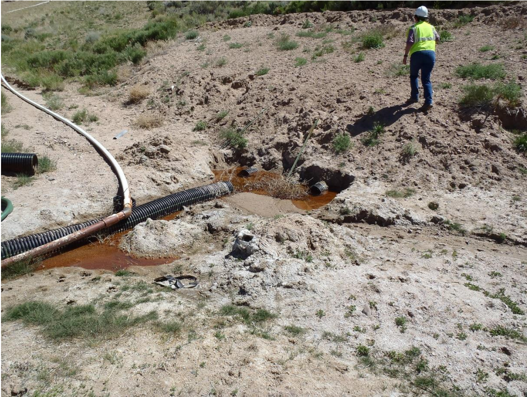
Photo 1. Three toe drain discharge pipes (manifold disconnected).
