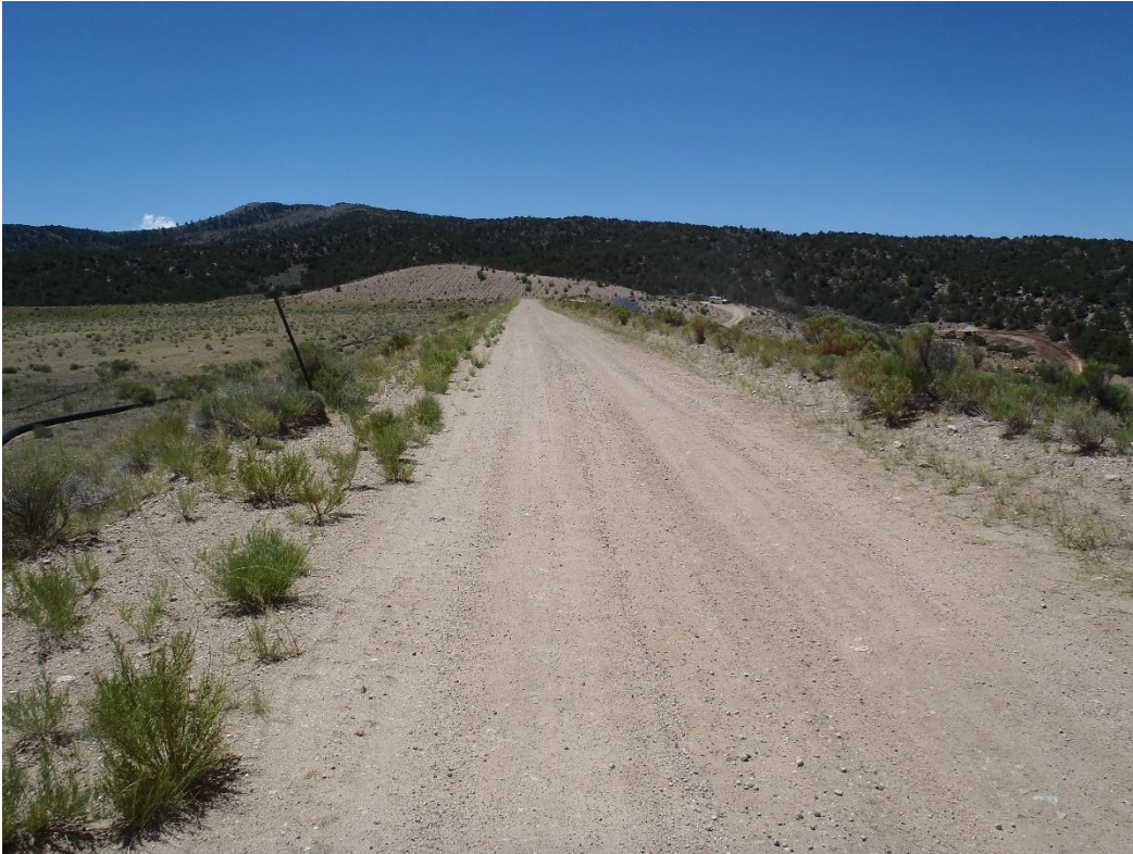
Photo 11. Dam crest (looking south from near center of dam crest).
