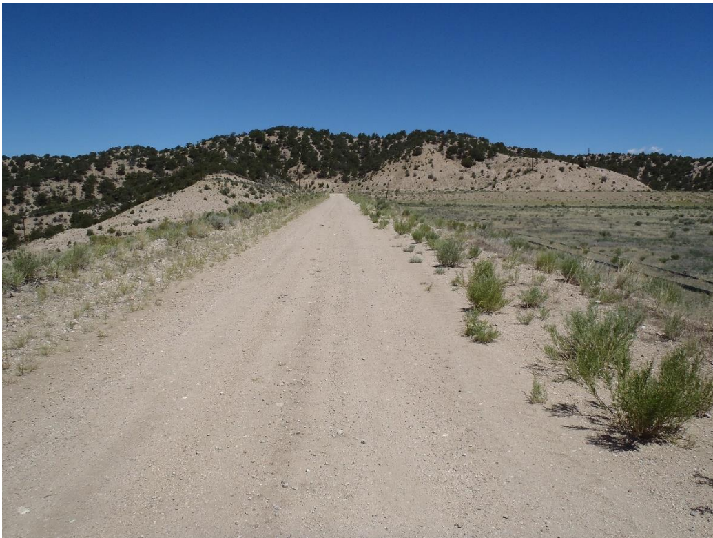
Photo 12. Dam crest (looking north from near center of dam crest).
