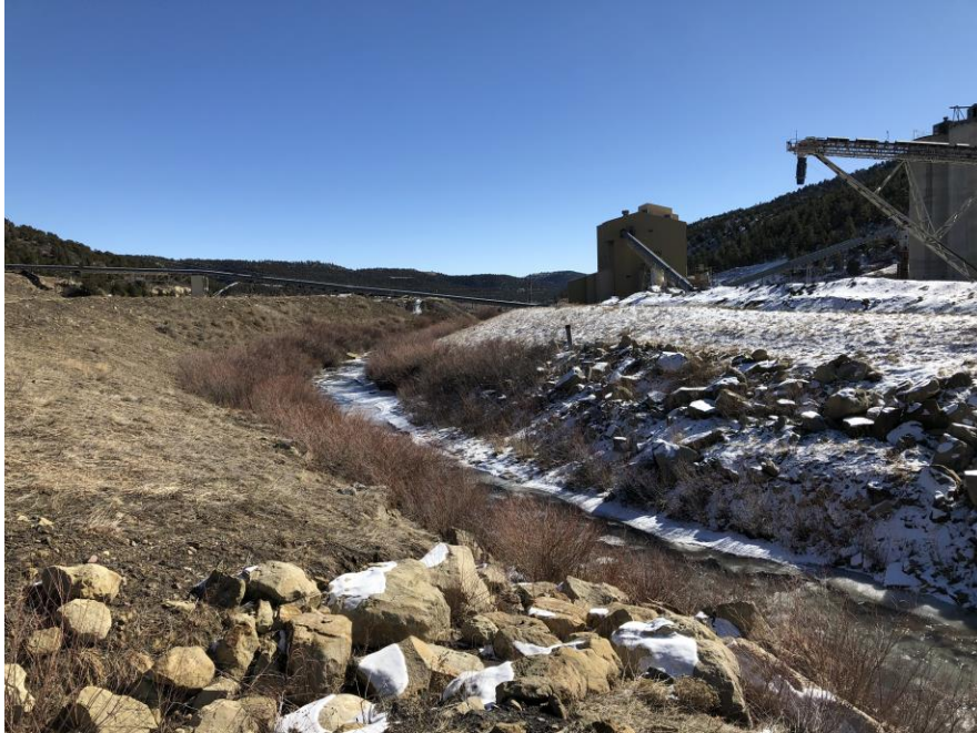
Riprap below SAE that is across Hwy 12 from Pond 08
