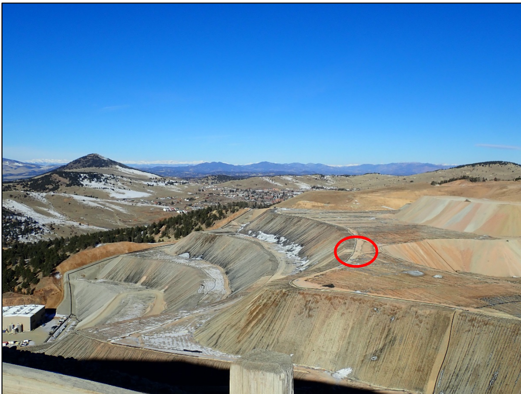
Photo 8. Washout on the 9,850' bench of the SGVLF bench circled in red; looking northwest.
