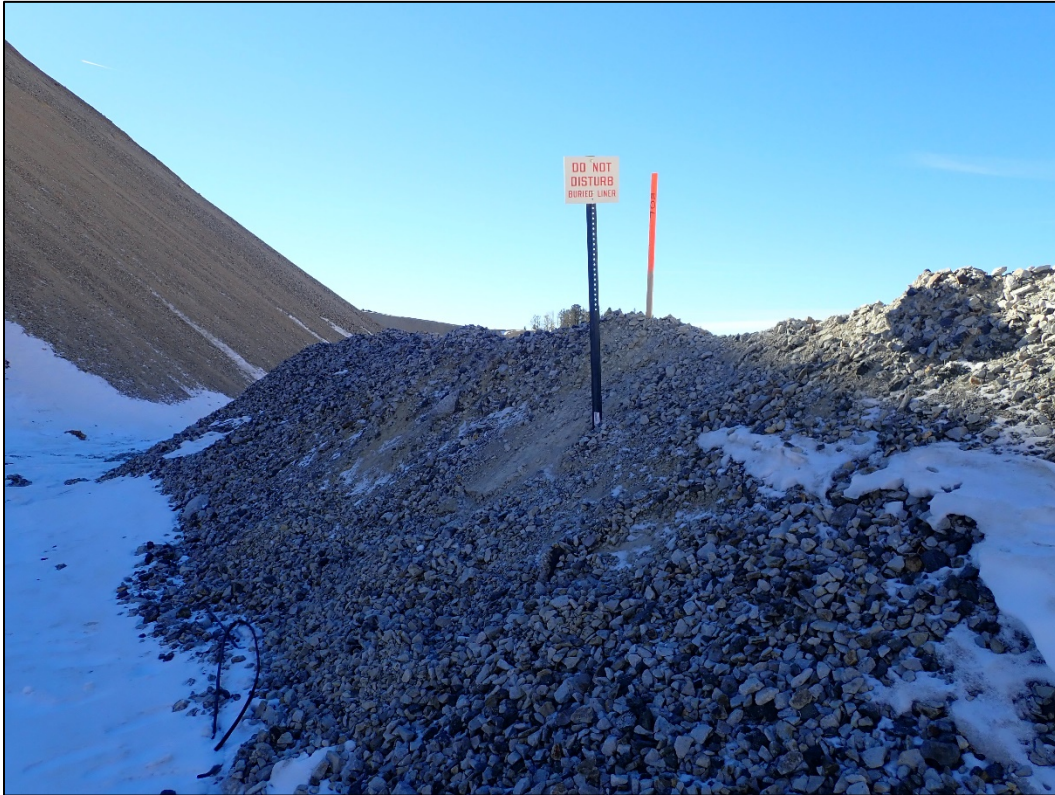
Photo 9. Recently installed Edge of Liner signs in the northwest portion of SGVLF; looking southwest.
