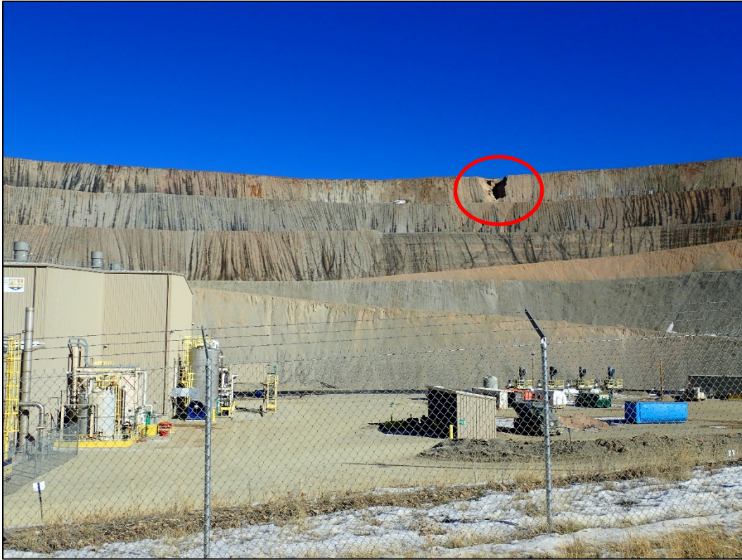
Photo 7. Washout on the 9,850' bench of the SGVLF bench circled in red; looking northeast from State Highway 67.
