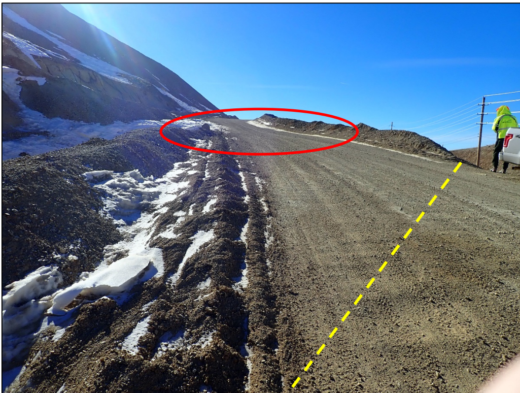
Photo 4. Access road in northwest portion of the AGVLF, edge of liner approximated by the dashed yellow line, area where storm water swale needs some work circled in red; looking south.
