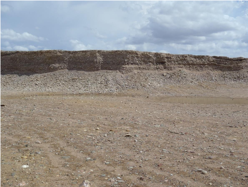
Photo 3. Typical highwall (south end).
