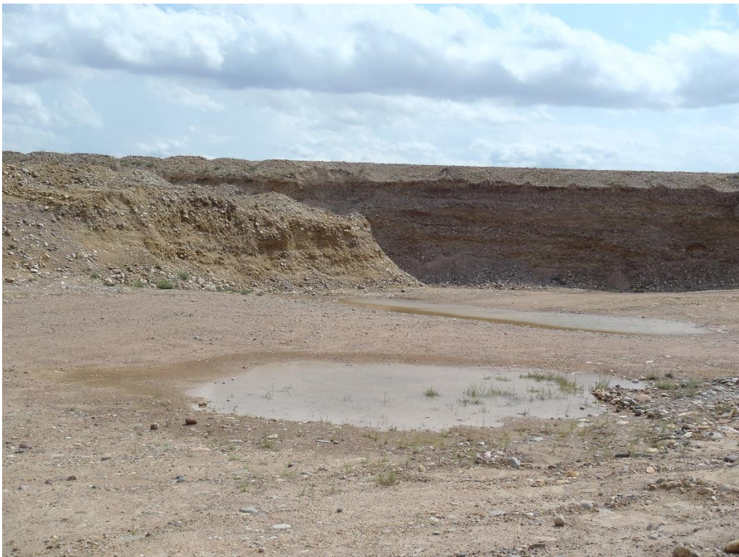
Photo 2. Puddles from recent rain in pit floor.
