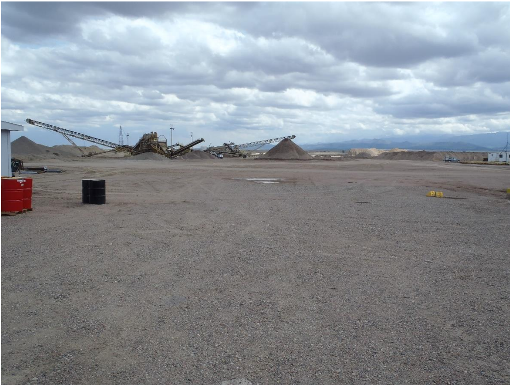
Photo 5. Screen plant (looking south, scale house on right).
