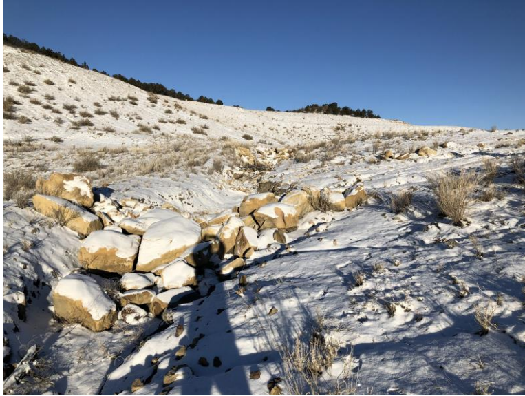
Ditch D9 with check dams
