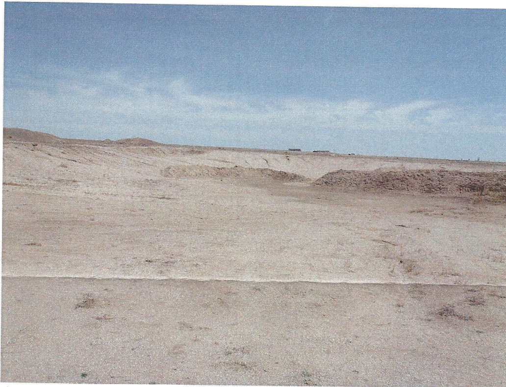
Photo 1. East (center background) and west (foreground) highwalls sloped at 5H:1V or flatter (looking NE).
