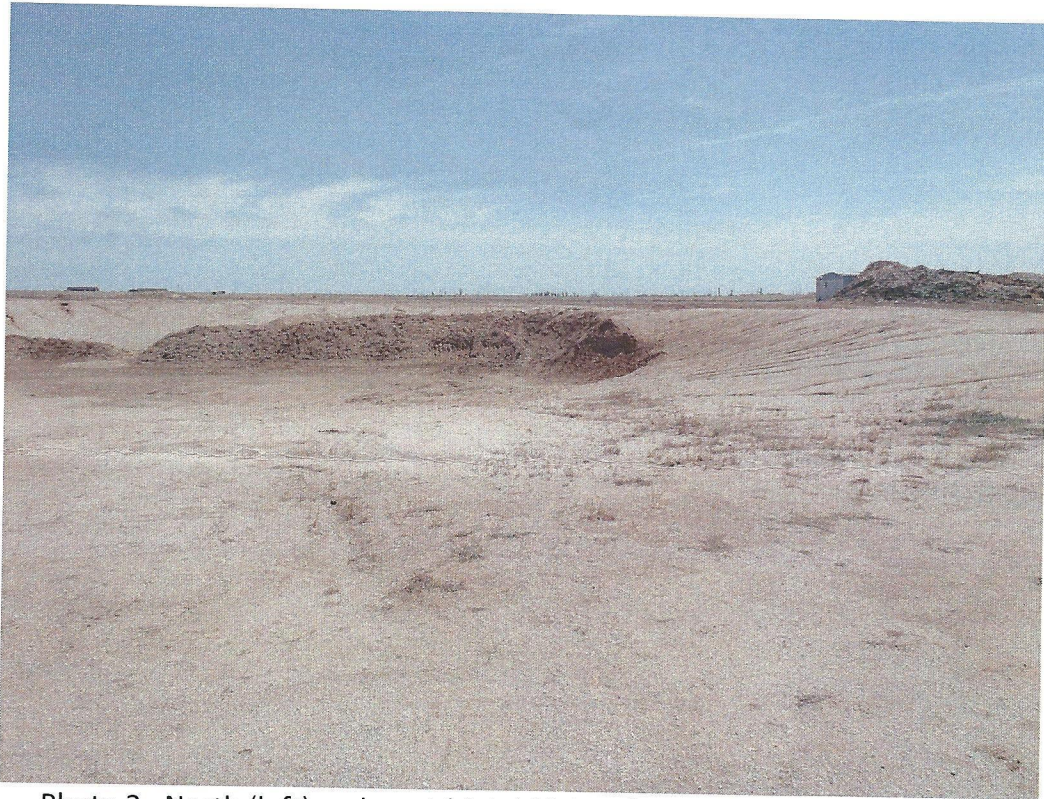
Photo 2. North (left) and west (right) highwalls sloped at 3H:1V or flatter.
