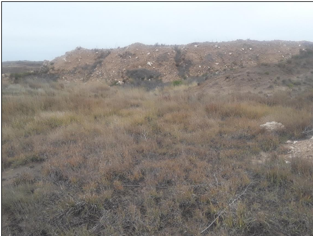
Photo 6. View looking west at overburden stockpile stored at eastern edge of active pit. Note stockpile is stable with some grass cover.
