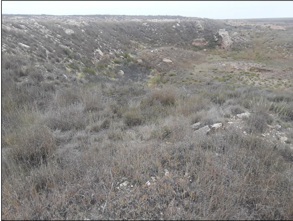
Photo 13. View looking northeast across old pit located west of active pit (in mining phases 4 and 6). Slope gradients in this area range from 1.5H:1V to 2.5H:1V. This area is well vegetated with volunteer grasses and shrubs, and appears to be stable.
