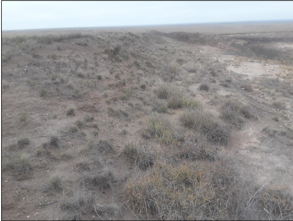
Photo 5. View looking south across topsoil stockpile stored at eastern edge of active pit. Note stockpile is stable with good grass cover.
