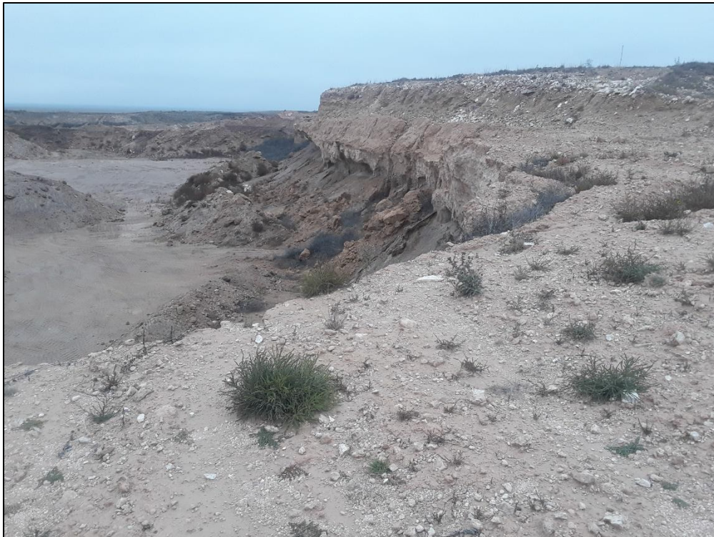
Photo 10. View looking west/southwest across portion of active highwall along northern edge of pit. Note erosion of softer substrate at bottom of highwall.
