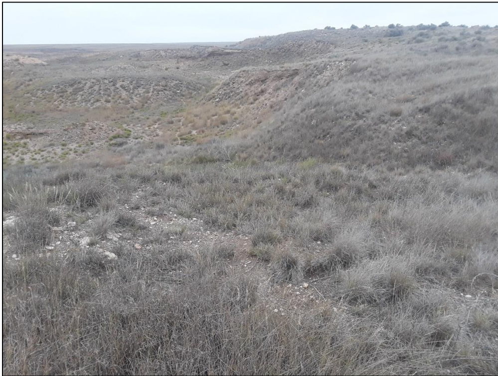
Photo 14. View looking southeast across old pit located west of active pit (in mining phases 4 and 6). Slope gradients in this area range from 1.5H:1V to 2.5H:1V. This area is well vegetated with volunteer grasses and shrubs, and appears to be stable.
