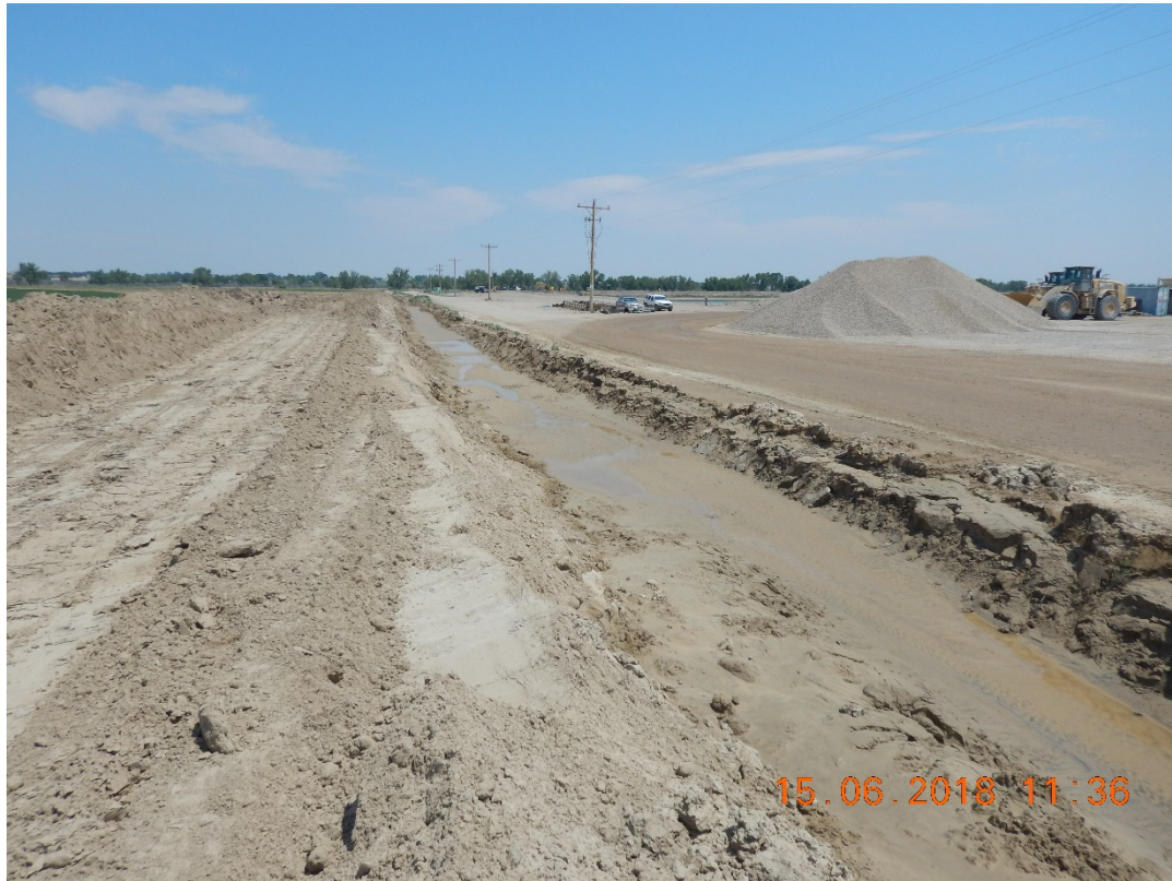
Photograph 5: Control measures not implemented along roadside ditch. Unauthorized process water and stormwater discharge location with a discharge of sediment to the Arkansas River.
