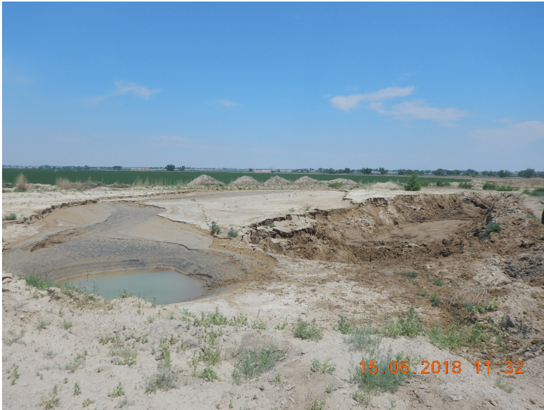
Photograph 15: Process water sediment ponds full of sediment and not maintained
