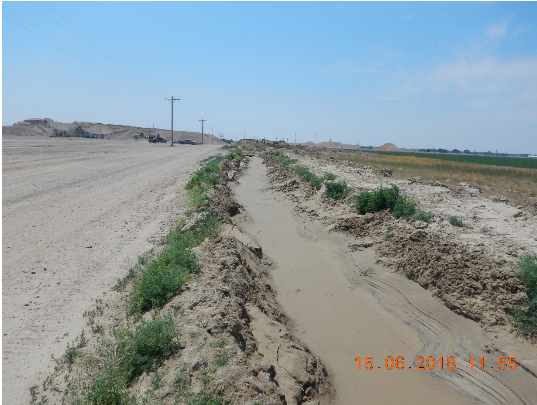
Photograph 7: Control measures not implemented along roadside ditch. Unauthorized process water and stormwater discharge location with a discharge of sediment to the Arkansas River.
