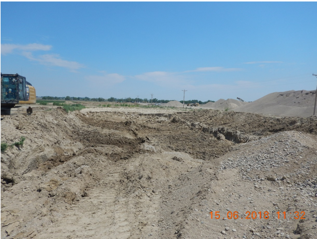
Photograph 14: Process water sediment ponds full of sediment and not maintained
