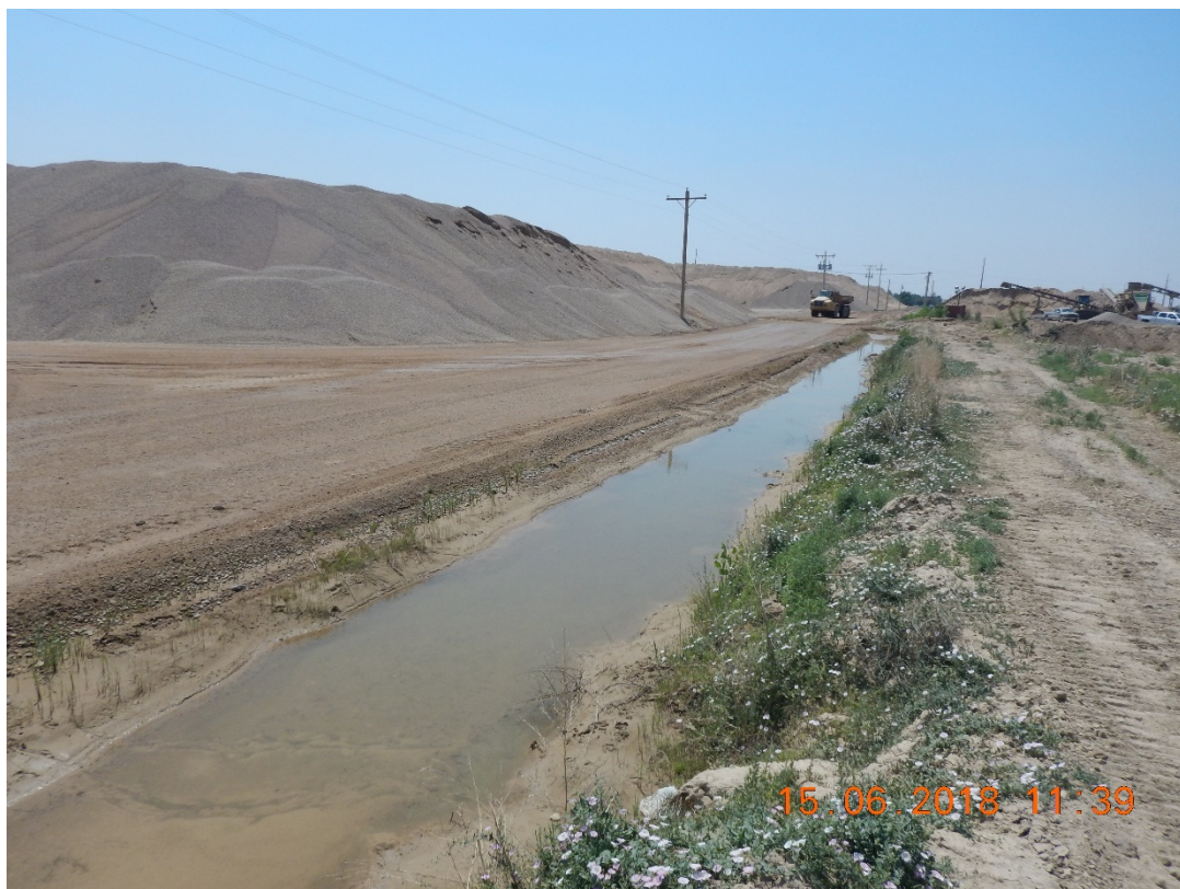
Photograph 4: Control measures not implemented along roadside ditch. Unauthorized process water and stormwater discharge location with a discharge of sediment to the Arkansas River.
