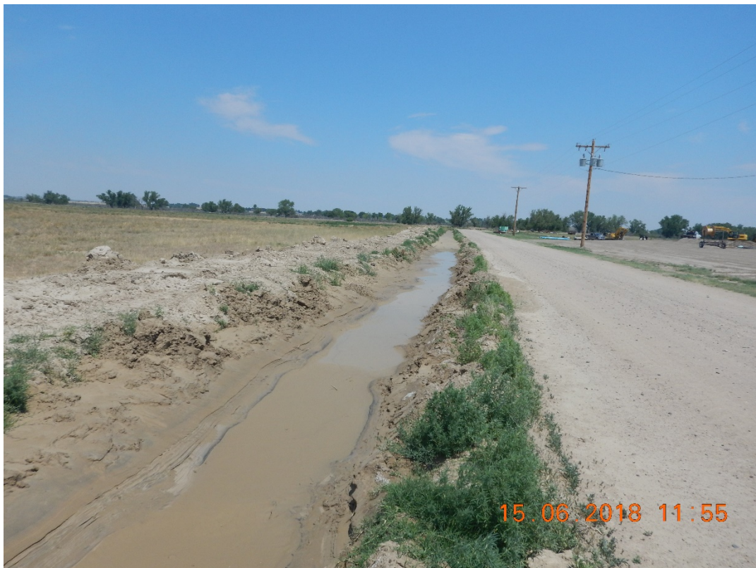
Photograph 8: Control measures not implemented along roadside ditch. Unauthorized process water and stormwater discharge location with a discharge of sediment to the Arkansas River.
