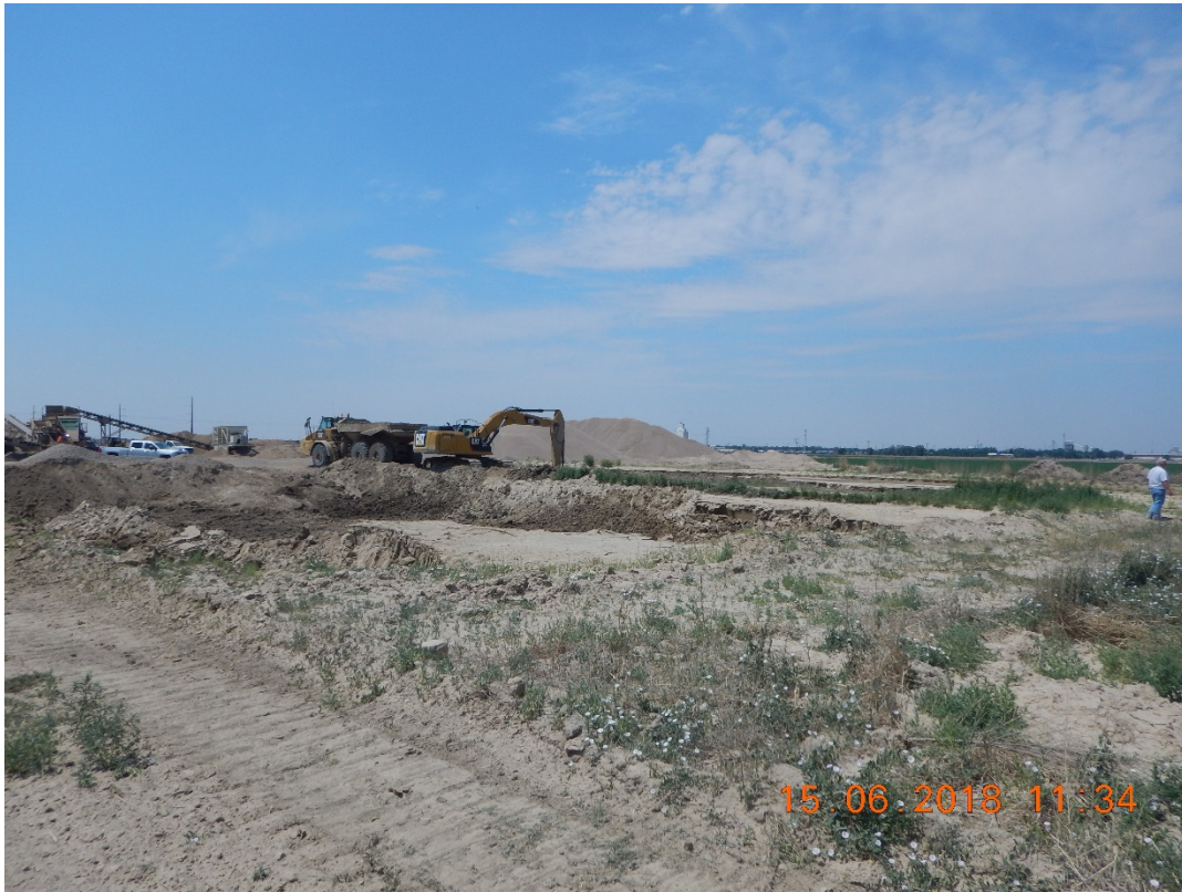
Photograph 17: Process water sediment ponds full of sediment and not maintained
