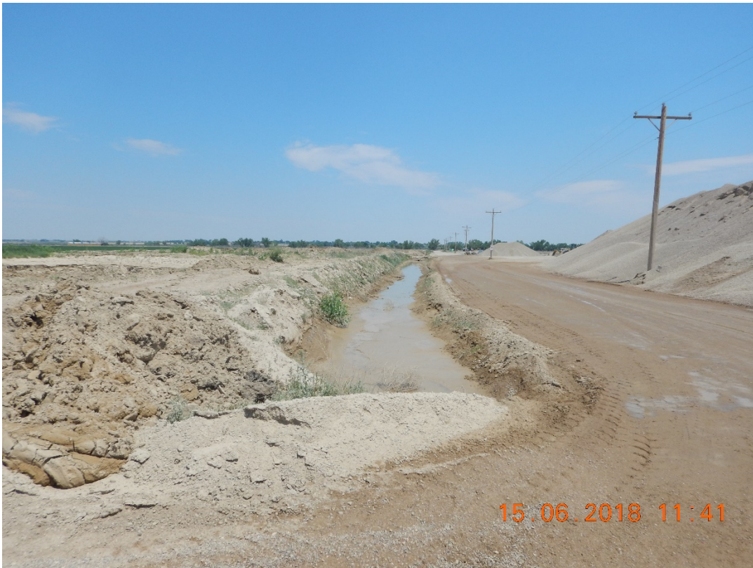
Photograph 6: Control measures not implemented along roadside ditch. Unauthorized process water and stormwater discharge location with a discharge of sediment to the Arkansas River.
