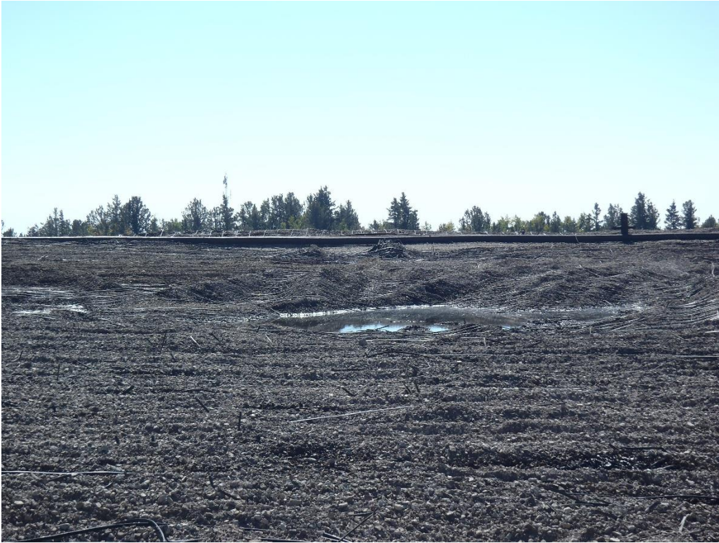
Photo 1. Ponded solution on VLF1 (10,400 level).
