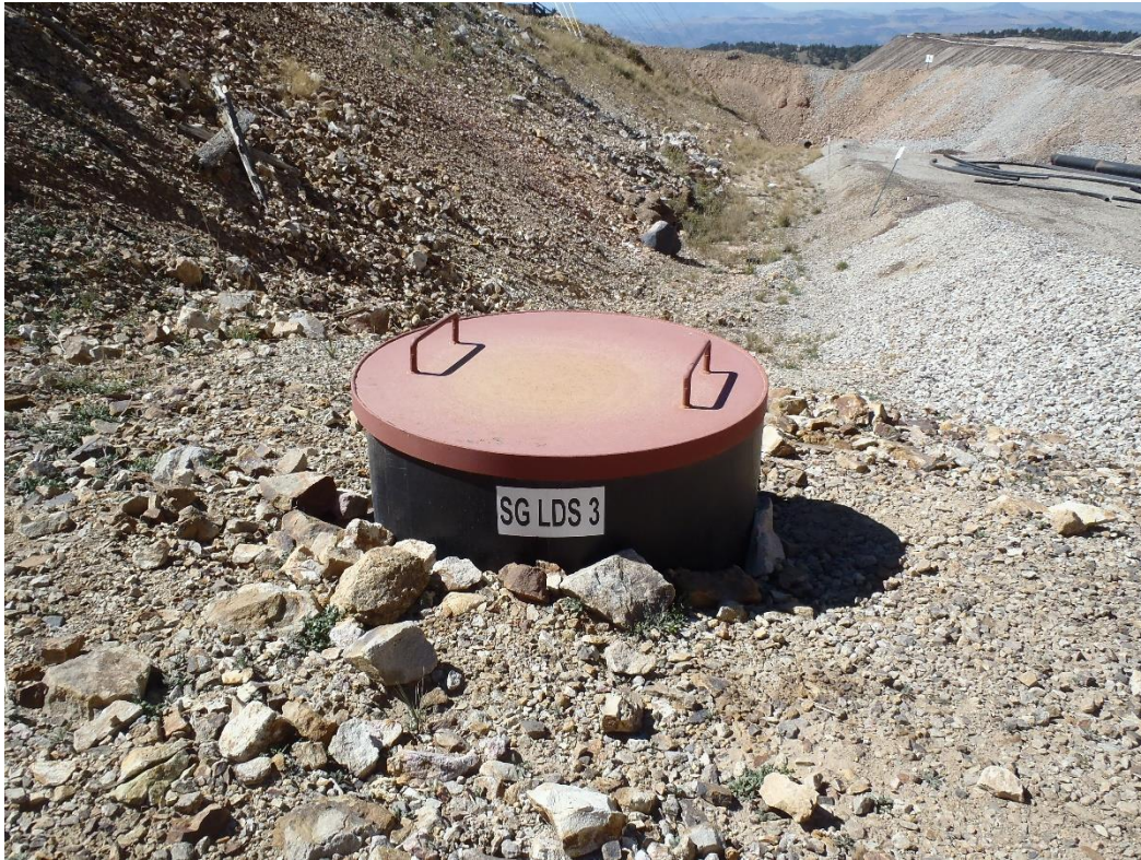
Photo 13. VLF2 LDS3 with adequate profile to prevent debris and meteoric water inflow.
