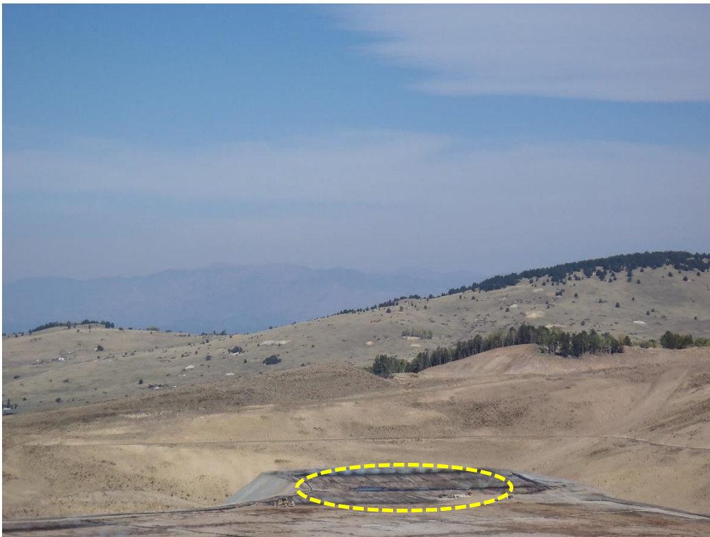
Photo 4. Ponded solution observed using binoculars on northwest side of VLF2 at the 9850 elevation.
