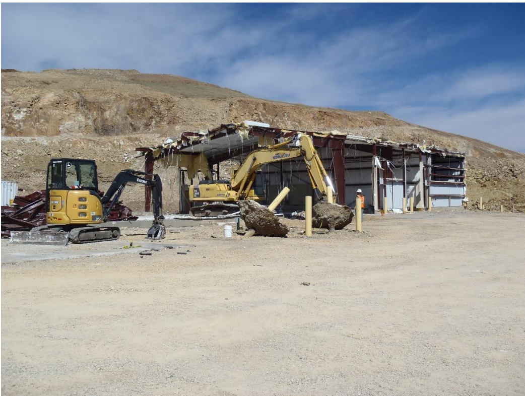
Photo 6. Demolishing the Ajax Building.
