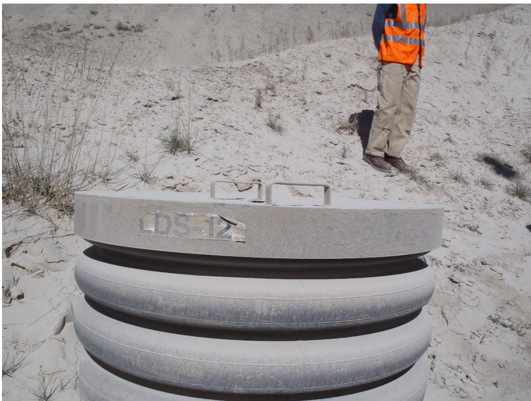
Photo 10. VLF1 LDS12 with adequate profile to prevent debris and meteoric water inflow.
