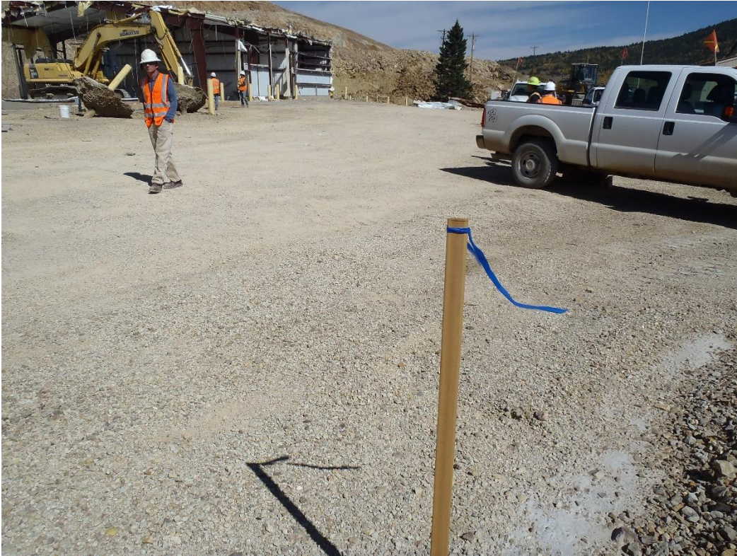
Photo 7. South Cresson pit limit staked with survey lathe.
