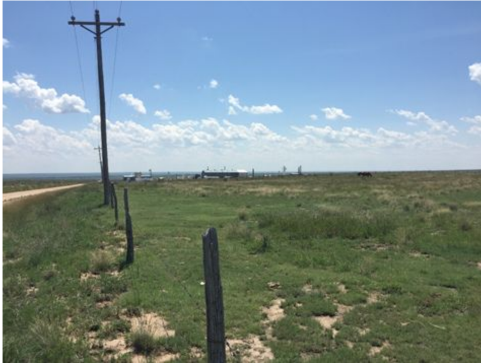
Photo 2 is a view of an oil and gas distribution site in Baca County proposal area.
