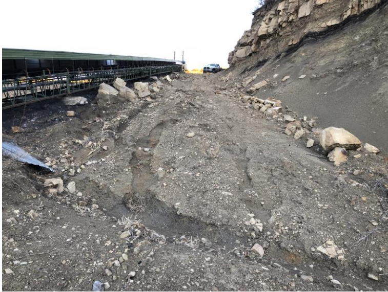
Eroding road next to conveyor
