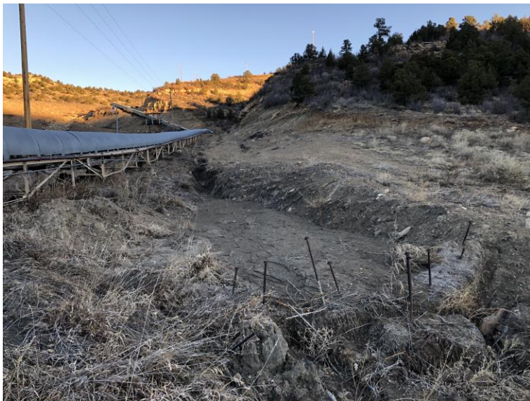
Eroding road next to conveyor with non-functioning sediment trap
