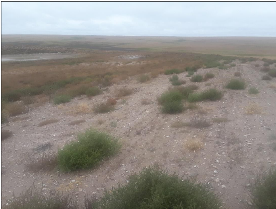
Photo 6. View looking east across southern pit slope which was graded to 3H:1V or flatter then seeded in November 2017. Vegetative cover of the pit area consists primarily of annual weeds at this time.
