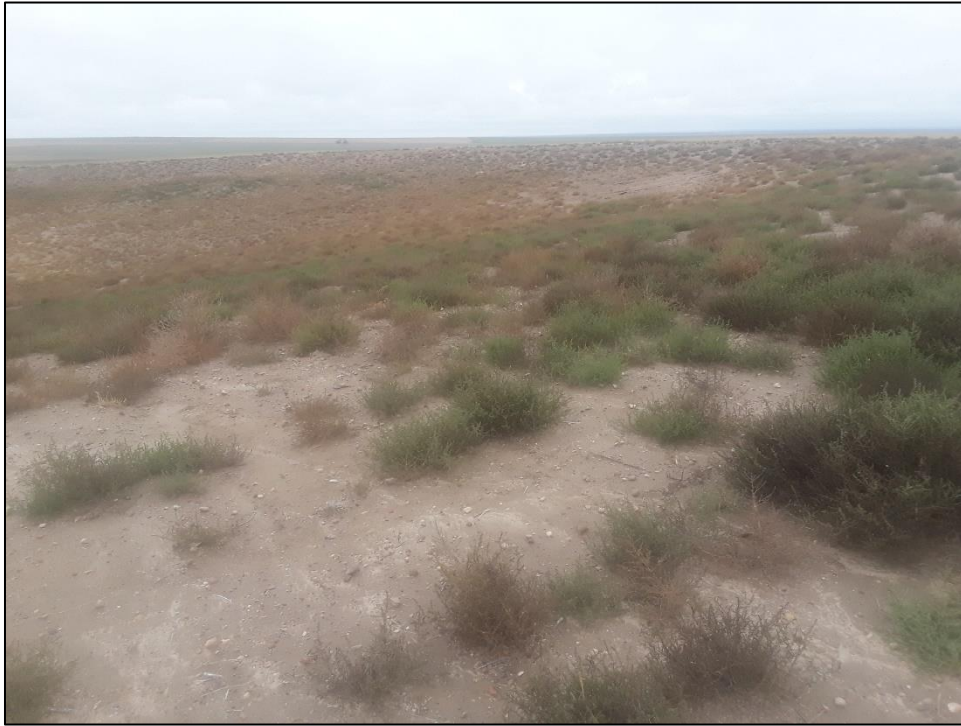
Photo 1. View looking south across western pit slope which was graded to 3H:1V or flatter then seeded in November 2017. Vegetative cover of the pit area consists primarily of annual weeds at this time.
