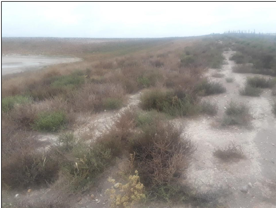
Photo 10. View looking west across northern pit slope which was graded to 3H:1V or flatter then seeded in November 2017. Vegetative cover of the pit area consists primarily of annual weeds at this time.
