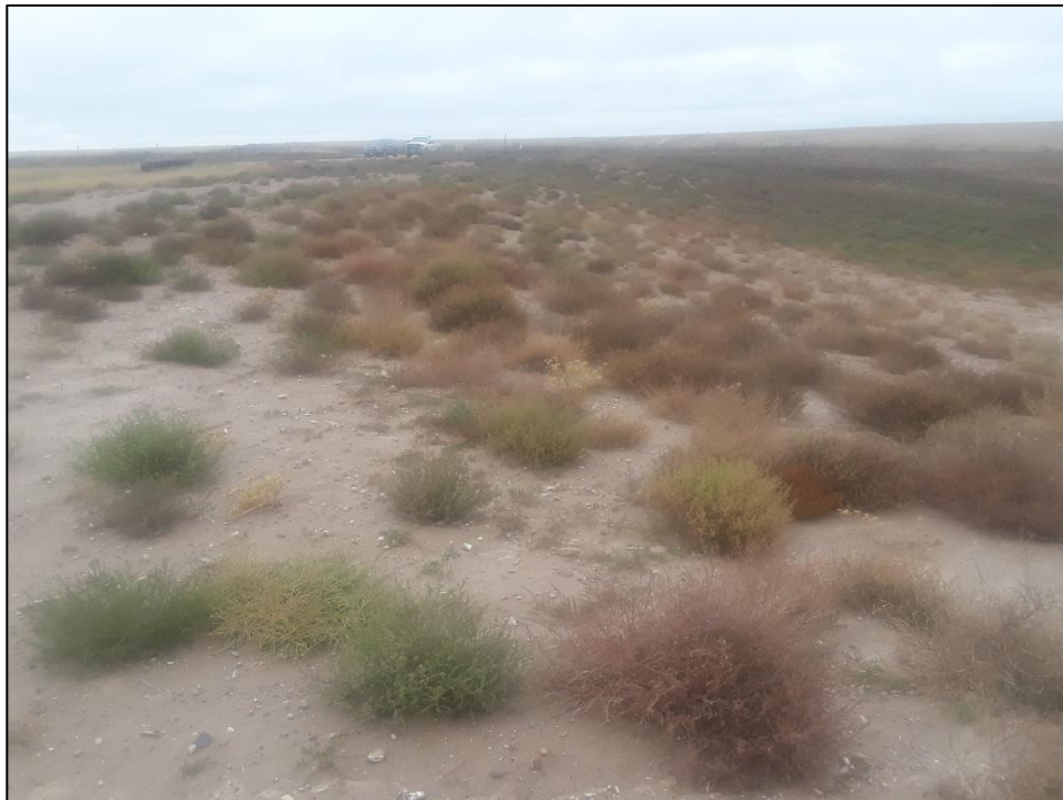
Photo 4. View looking north across western pit slope which was graded to 3H:1V or flatter then seeded in November 2017. Vegetative cover of the pit area consists primarily of annual weeds at this time.
