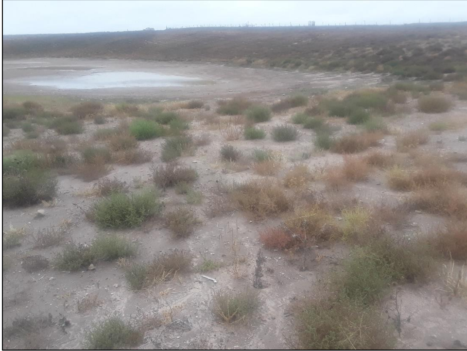
Photo 9. View looking northwest across pit from its eastern edge. Note eastern pit slope (shown in foreground) is graded to flatter than 3H:1V.
