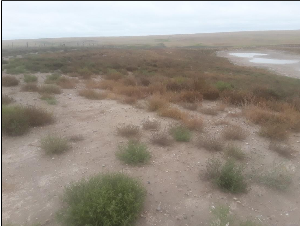
Photo 3. View looking east across northern pit slope which was graded to 3H:1V or flatter then seeded in November 2017. Vegetative cover of the pit area consists primarily of annual weeds at this time.
