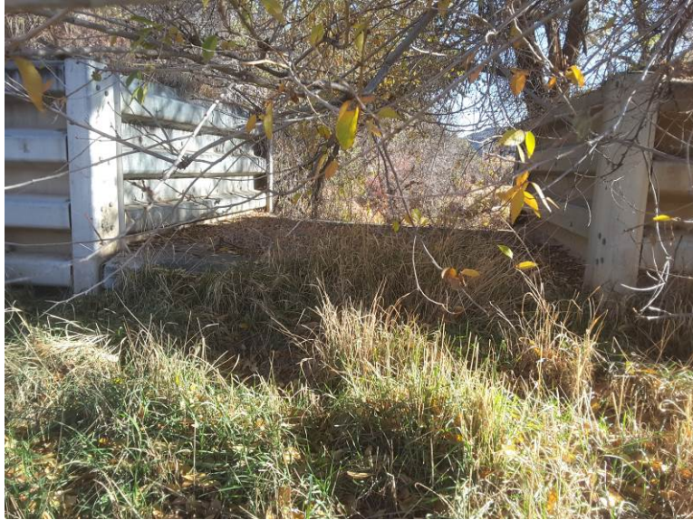
Figure 6. Unobstructed principal spillway, Loadout Pond.
