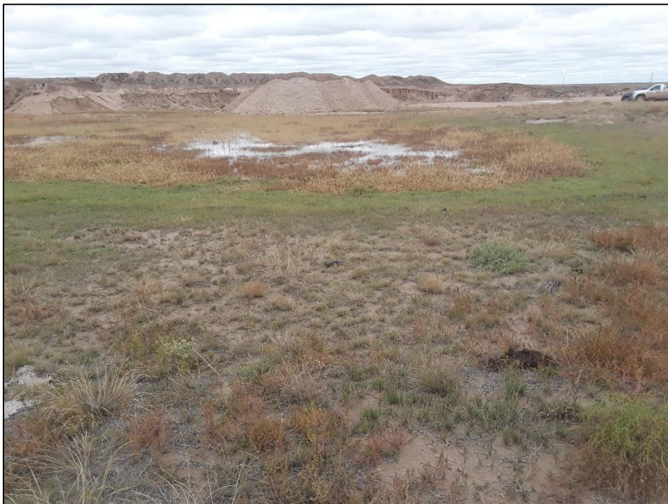
Photo 8. View looking north across reclaimed southern portion of site. Slopes are graded to 3H:1V or flatter. Vegetative cover consists of native grasses, forbs, and annual weeds. (Active mining area visible in background)
