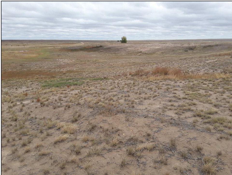
Photo 10. View looking southeast across reclaimed southern portion of site. Slopes are graded to 3H:1V or flatter. Vegetative cover consists of native grasses, forbs, and annual weeds. Some portions of slopes may need to be reseeded.
