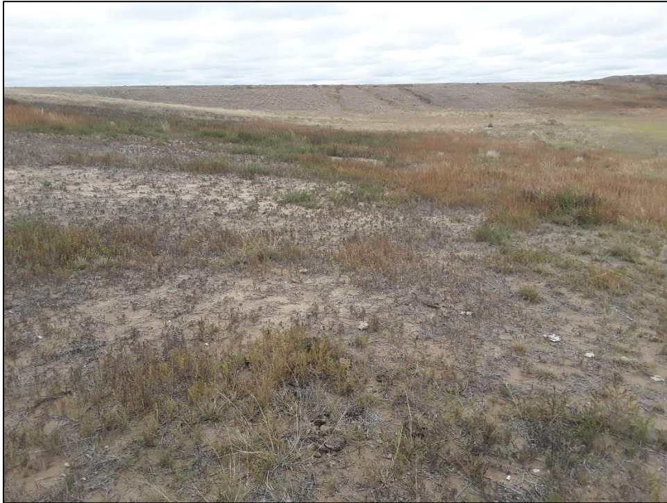
Photo 7. View looking northwest across reclaimed southern portion of site. Slopes are graded to 3H:1V or flatter. Vegetative cover consists of native grasses, forbs, and annual weeds. Some portions of slopes may need to be reseeded.
