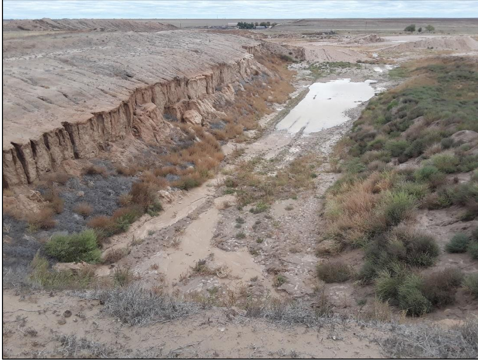
Photo 3. View looking east across active pit from its western edge. Note pit floor holding some water during inspection due to recent storm event.
