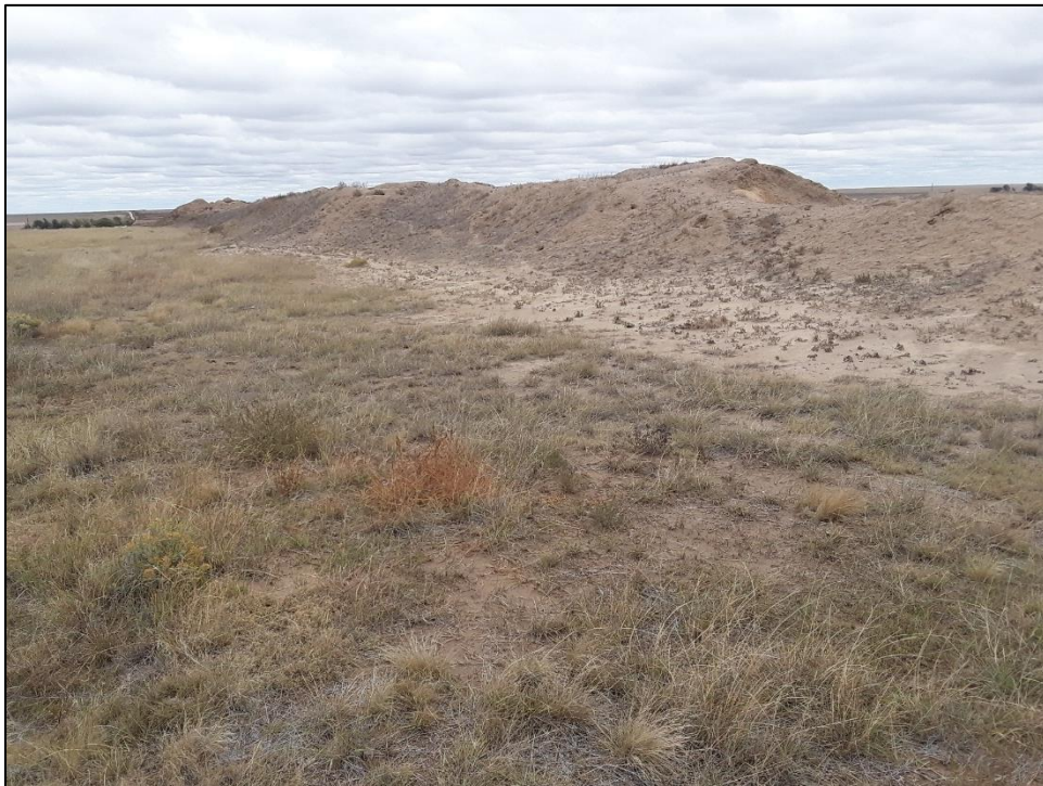
Photo 6. View looking southeast at topsoil stockpile stored along northern permit boundary, which appeared to be stable with some vegetative cover.
