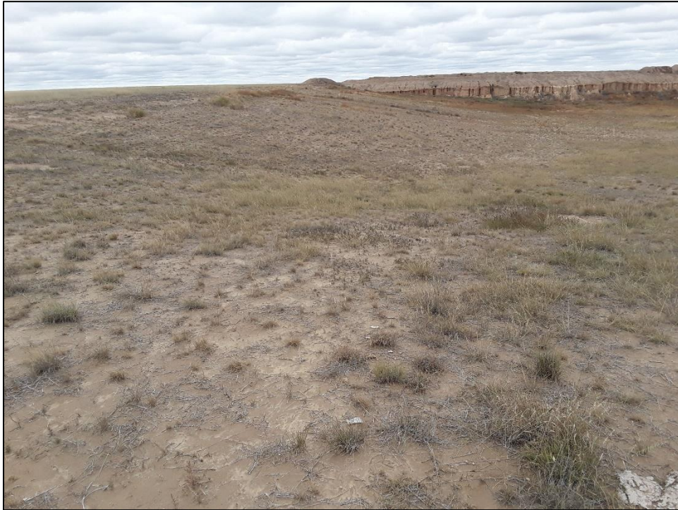
Photo 9. View looking north across western reclaimed highwall. Slopes are graded to 3H:1V or flatter. Vegetative cover consists of native grasses, forbs, and annual weeds. Some portions of slopes may need to be reseeded.
