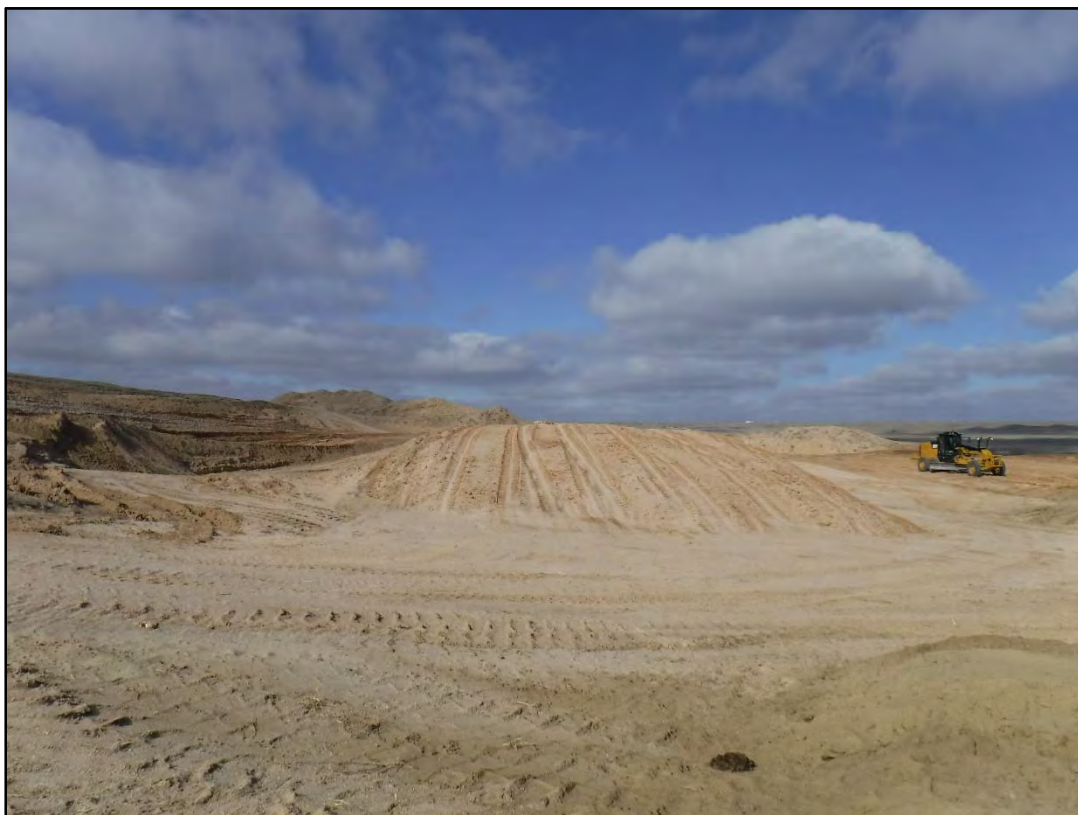
Photo 6: Recently placed stockpile of material to be blended with import material.
