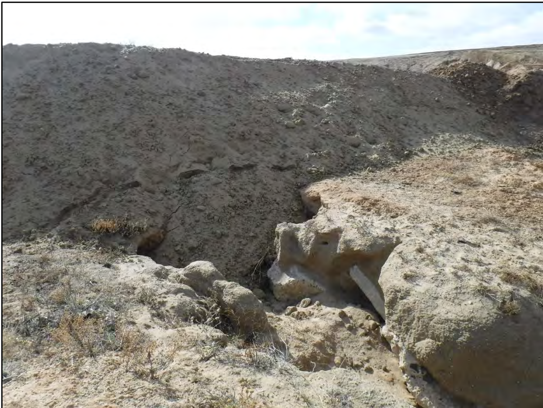
Photo 4: Berm across drainage to prevent off site damage.
