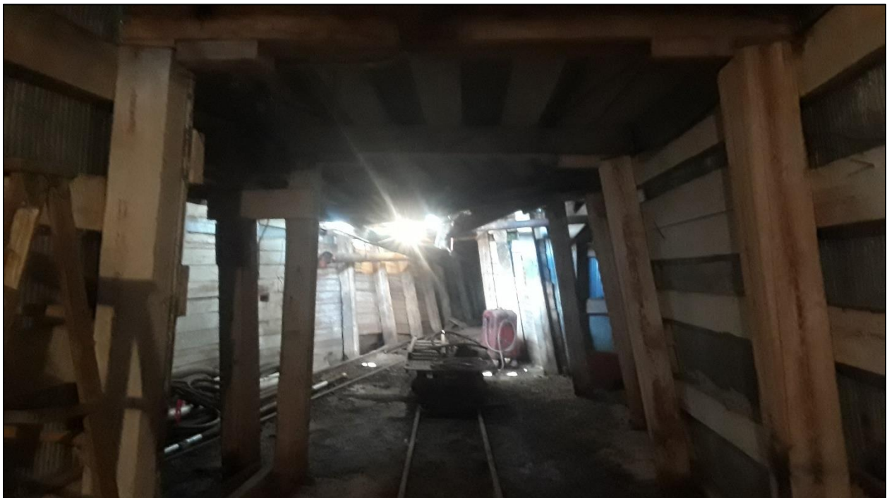
Photo 24. View inside of Caribou Mine snowshed which was constructed with timbers in the 1940's. This snowshed will require rehabilitation prior to using it to access the Caribou Mine/Idaho Tunnel.
