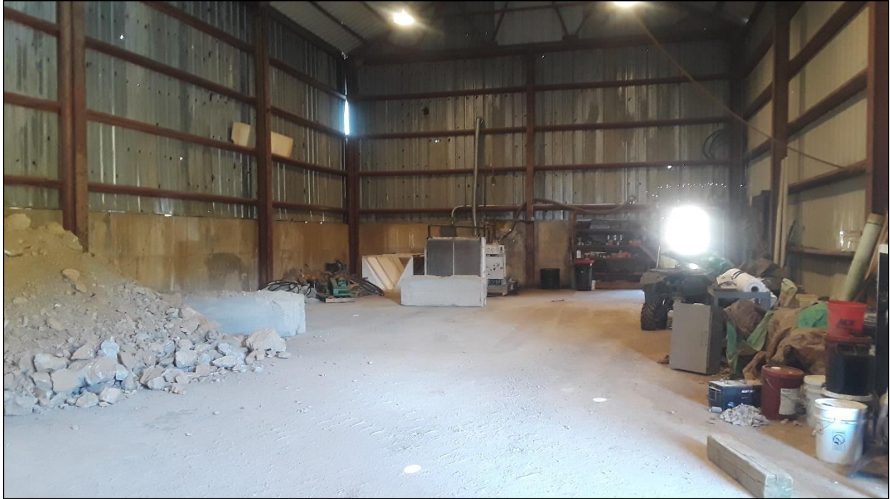
Photo 7. View inside Cross Mine warehouse which has thick concrete floors and retaining walls.
