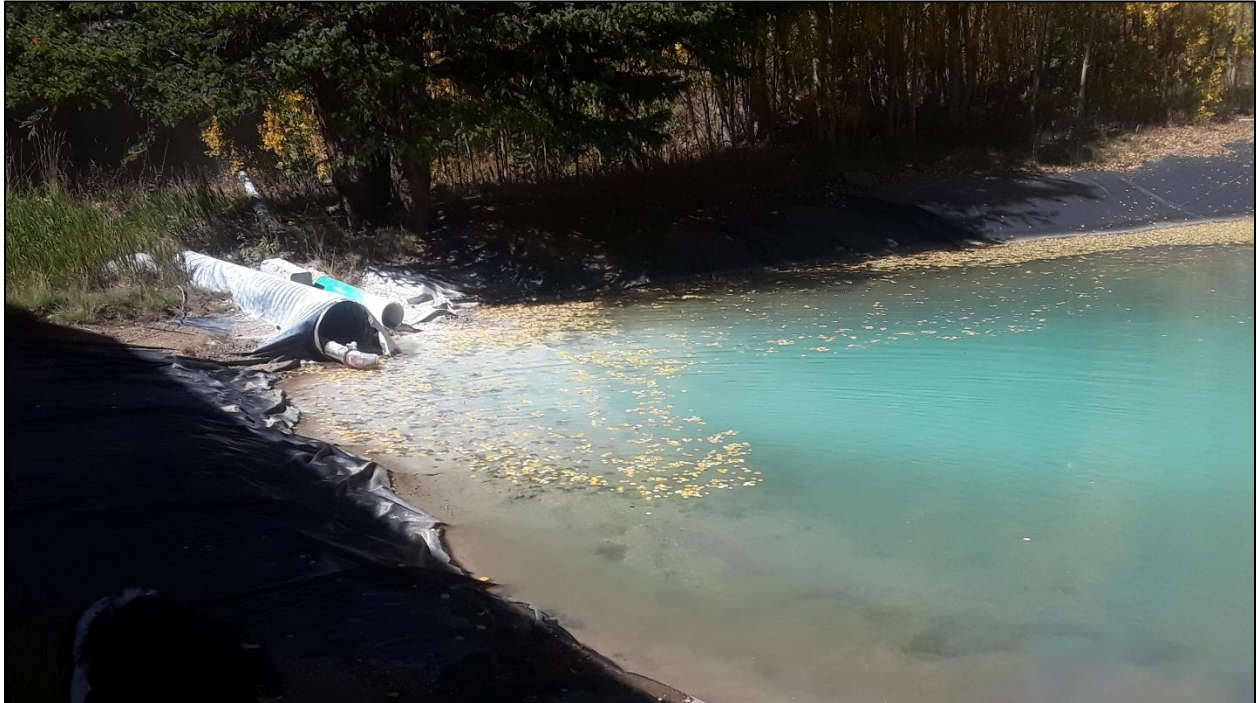
Photo 14. View of western edge of pond #1 where Cross Mine water discharges to pond via pipeline. This water is treated with lime on a daily basis in accordance with the NPDES permit.
