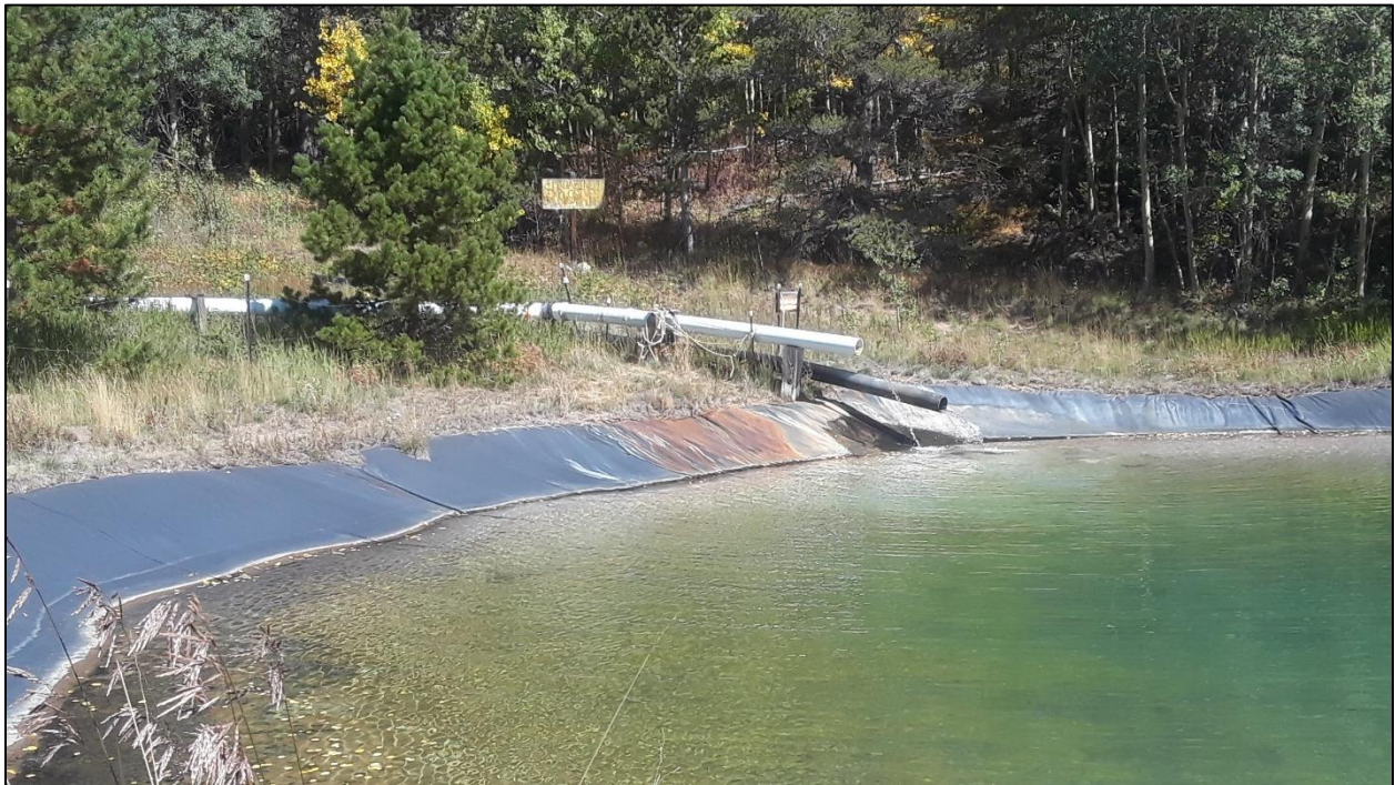
Photo 16. View of northern edge of pond #2 where mine water is discharged to pond via pipeline at a combined rate of approximately 45-50 gpm (white pipeline = Cross Mine water, black pipeline = Caribou Mine water).
