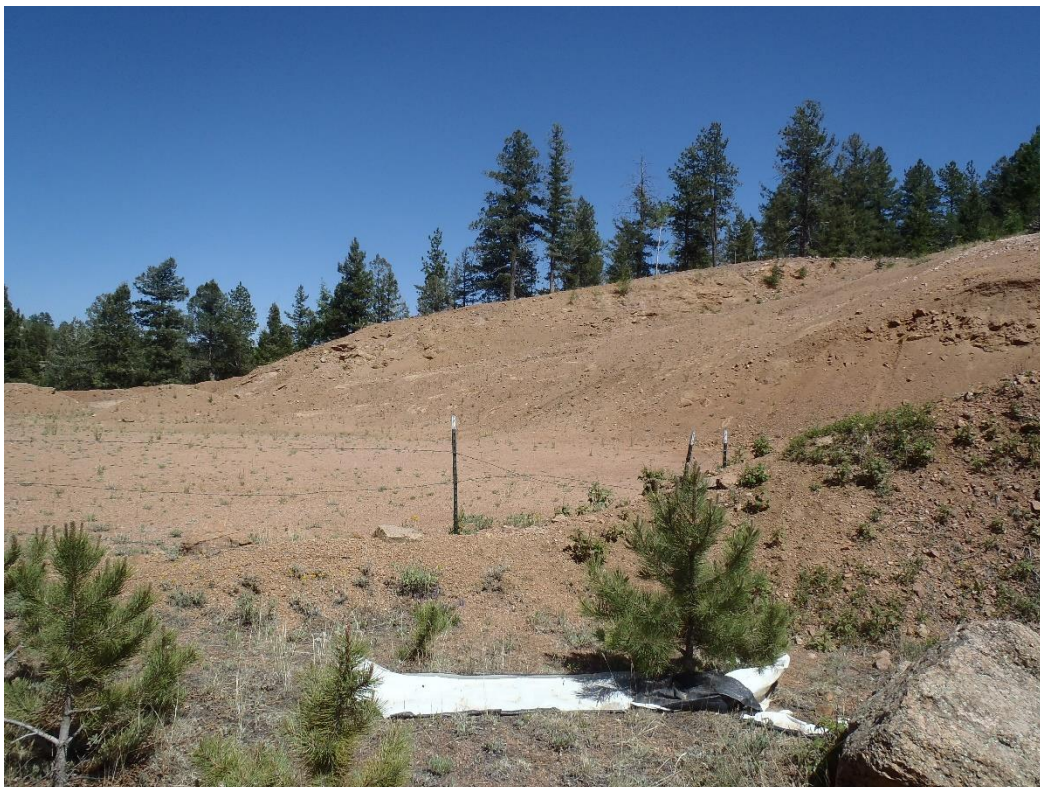
Photo 3. Active highwall (~2.5H:1V, looking east, note fence marking west boundary).
