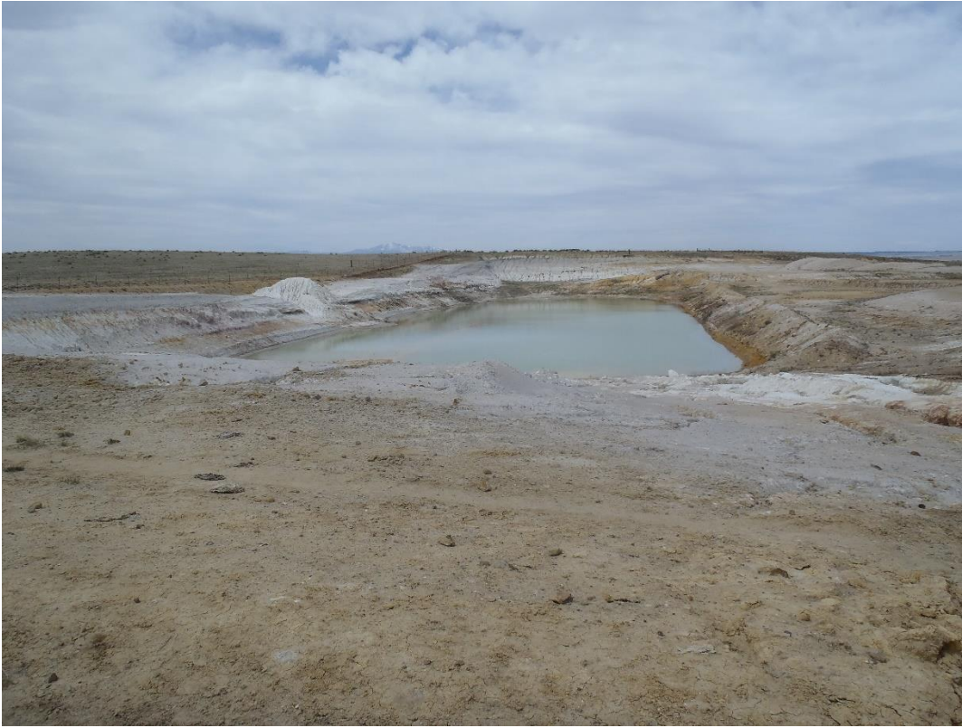
Photo 1. Probable exposed groundwater observed in the south pit of Stage 1A (looking west).
