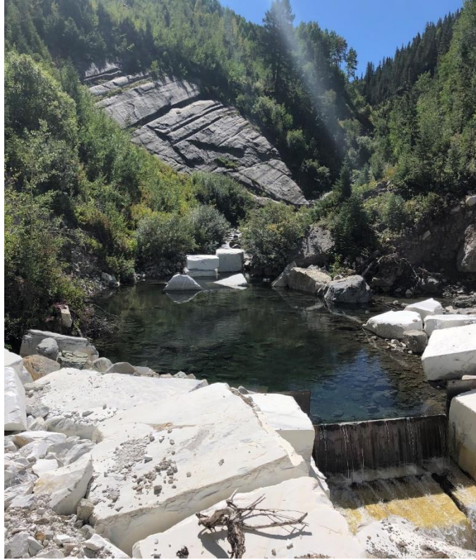
Figure 3. Example ‘pond’ structure of Yule creek just upstream of the point of diversion. Installation of porous weirs along the diversion will serve the same purpose as the metal weir in this image – to slow water flow and allow time and space for sediment to settle out of suspension. Installed weir is part of a flow monitoring for a potential hydro power project. View to the south. Photo captured: 180830.
