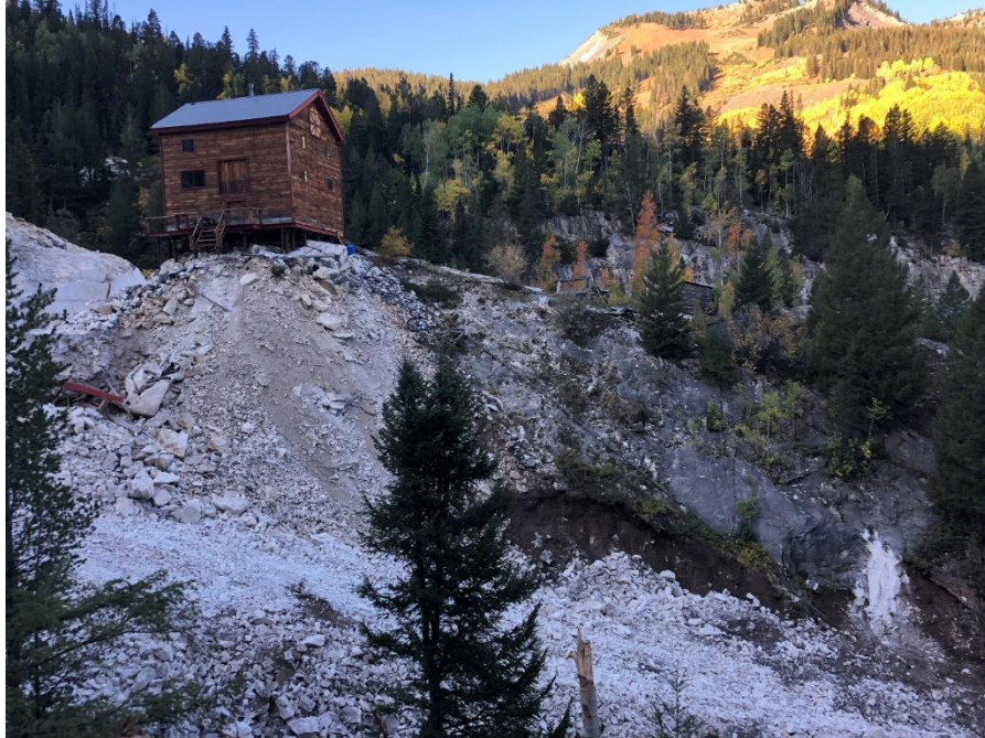
Figure 2. Current state of the diversion approximately 1,000 feet from the point of diversion. Notice the abundance of marble rubble and exposed bedrock (grey cliff forming member) with minor soil and debris. View to the west. Photo captured 180918.
