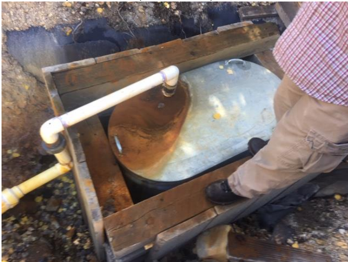
Slag treatment system inlet.
