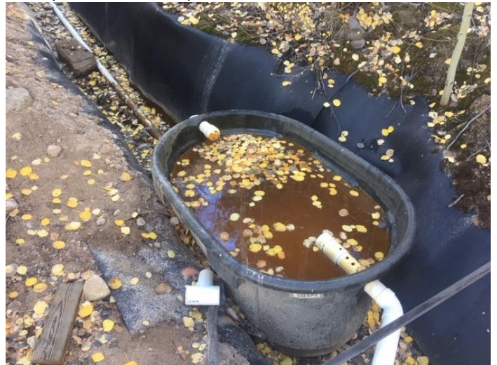
Treatment system settling point.
