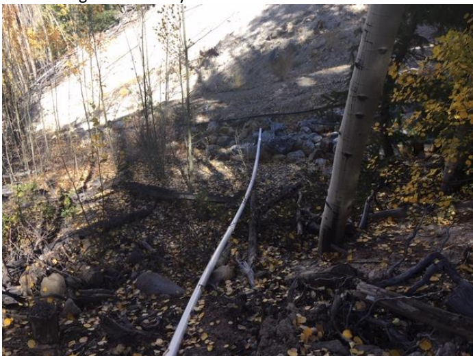
Treatment system outlet into limestone channel.
