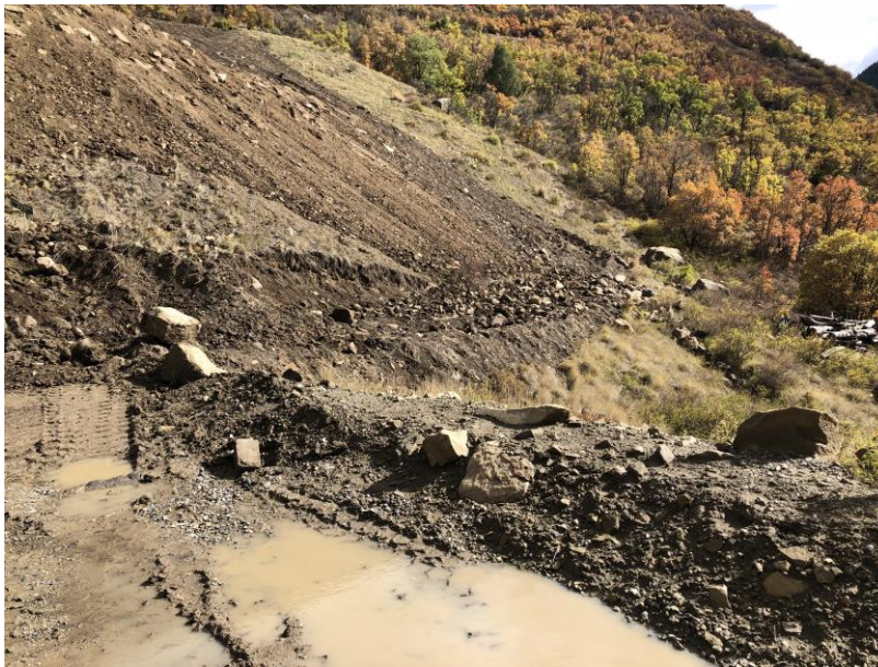
Ditch below topsoil stockpile (at Upper Elk Creek Pad) needs to be cleared of soil
