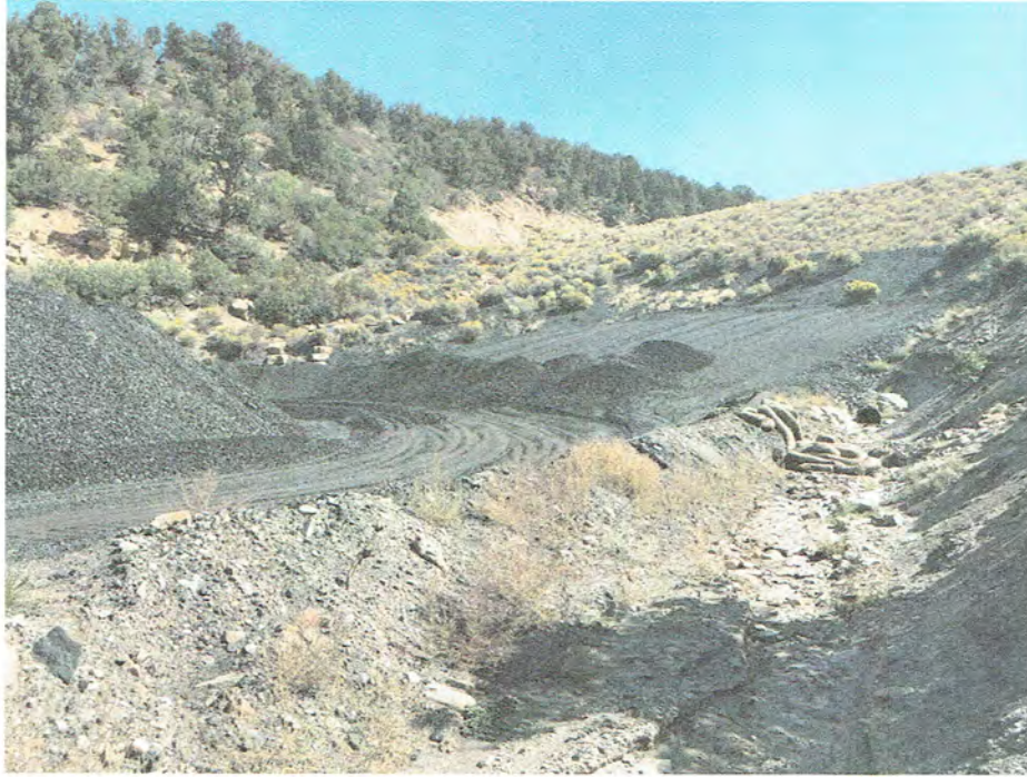
Pic. 5 – Additional material placed at base of embankment.
