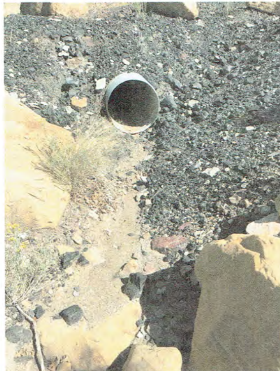
Pic. 2 – Culvert under haul road for south ditch.
