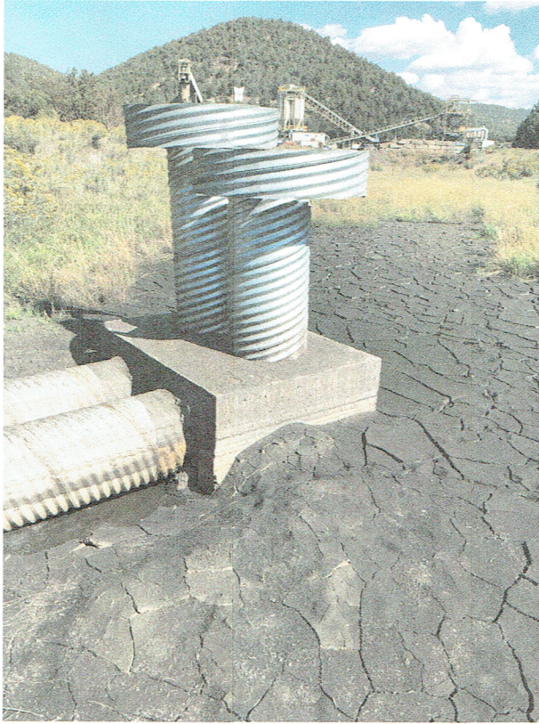
Pic. 1 – Detention Pond outlet structure, dry.
