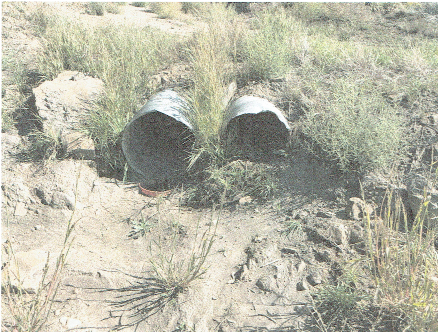
Pic. 2 – Dual culverts from outlet structure in good condition.
