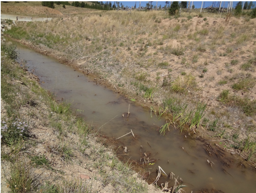
View of mechanically removed cattails in the ultimate canal
