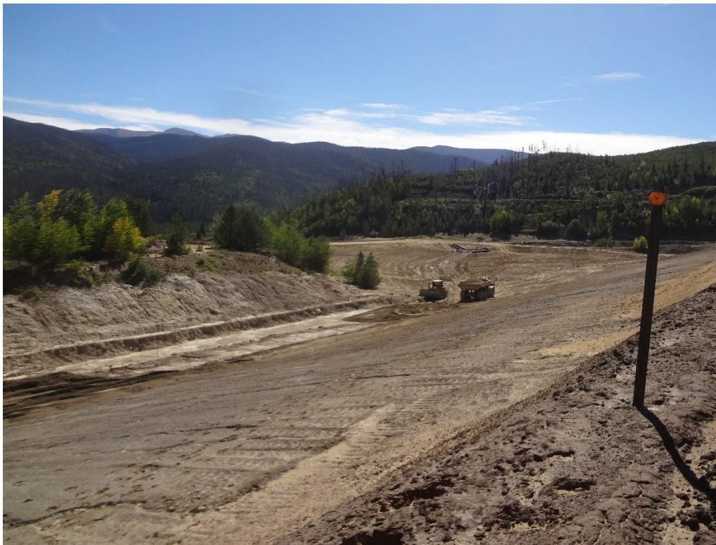
View of filter sand placement on the south side of the 3-Dam stepback looking south
