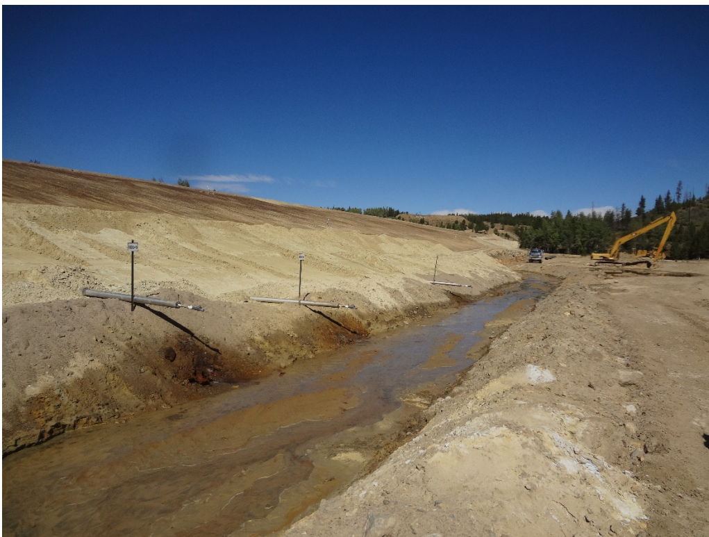
View of extended toe drains at the south toe of 3-Dam
