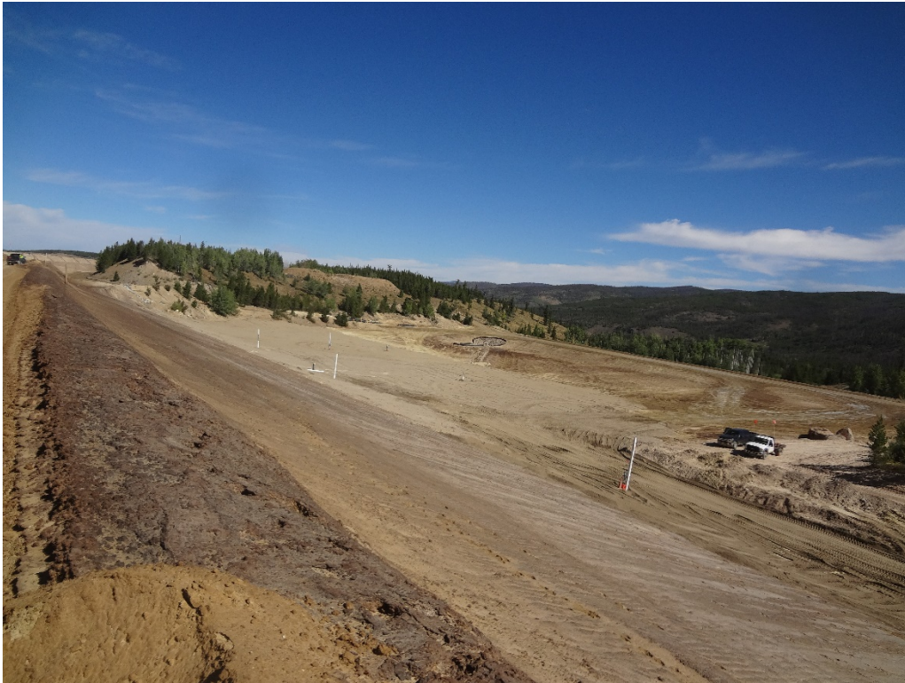
View of completed filter sand placement on the north side of the 3-Dam stepback looking north
