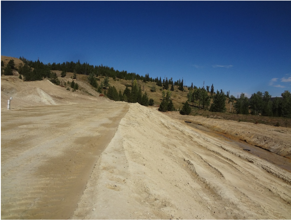
View of completed tailings sand placement at the north toe of 3-Dam
