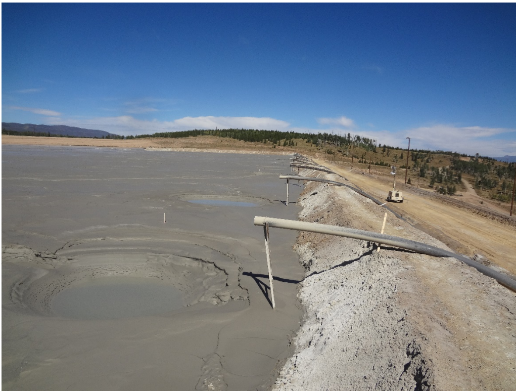
View of tailings deposition in Cell 8 of 1-Dam looking north
