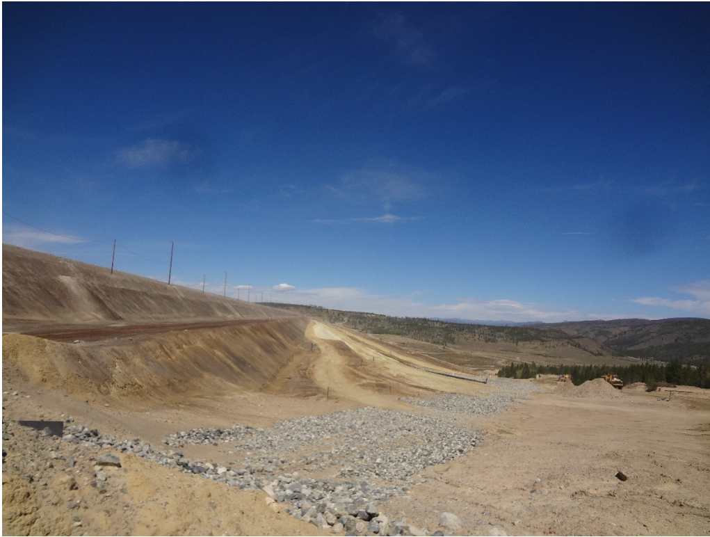
View of the removal of the inter-benches on 1-Dam
