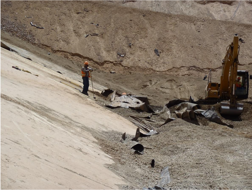
Photo 1. Bottom of VLF 2 liner damage still being uncovered (near 9650 bench).
