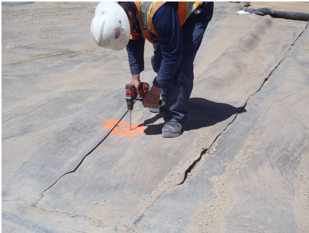
Photo 4. Checking soil liner fill (SLF/"clay") thickness.
