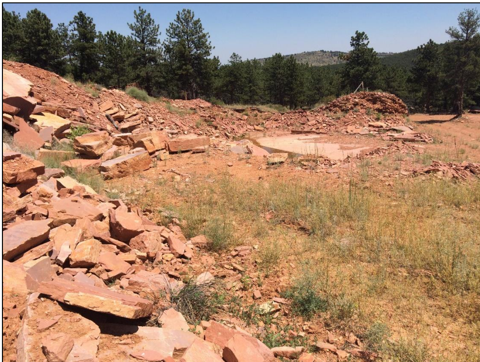
Photo 2. View looking east across south pit area. Loose rocks will need to be pushed into pit and graded out to 3H:1V or flatter for reclamation.
