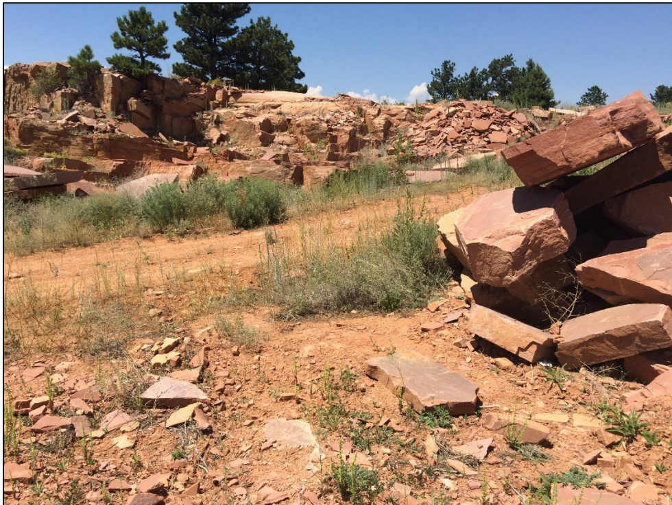
Photo 4. View looking west across south pit area. Loose rocks will need to be pushed into pit and graded out to 3H:1V or flatter for reclamation. Mine walls will need to be graded to 3H:1V or flatter.
