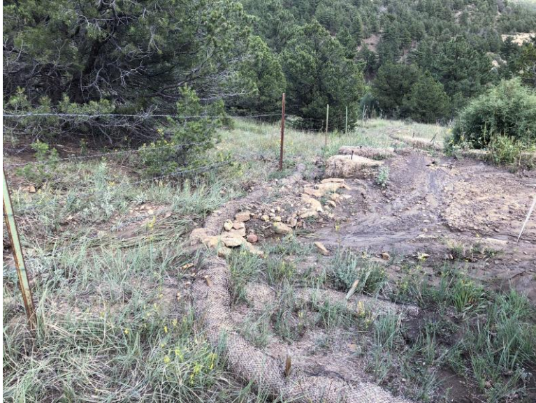
Erosion BMPs in need of maintenance at old North Shaft site
