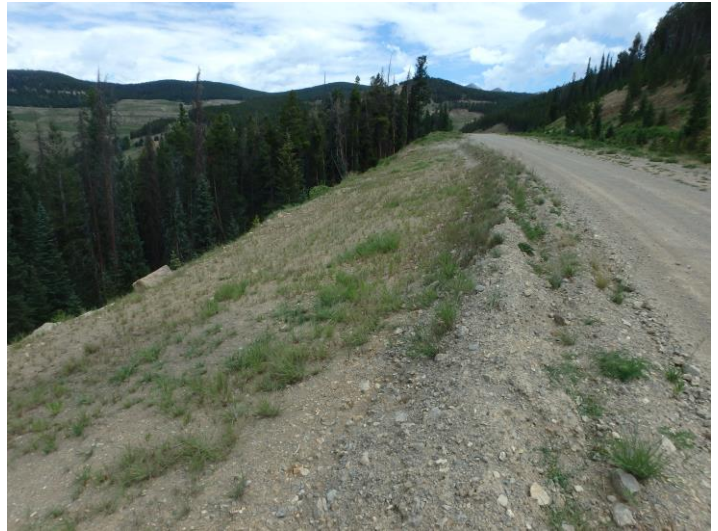
Repaired slough area on access road
