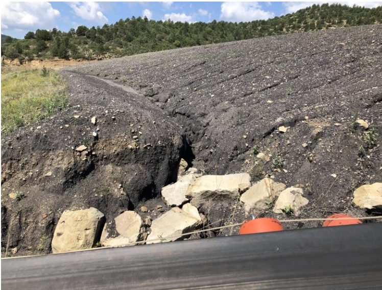
Interface of upper and lower portions of RDA - East side where additional riprap should be placed
