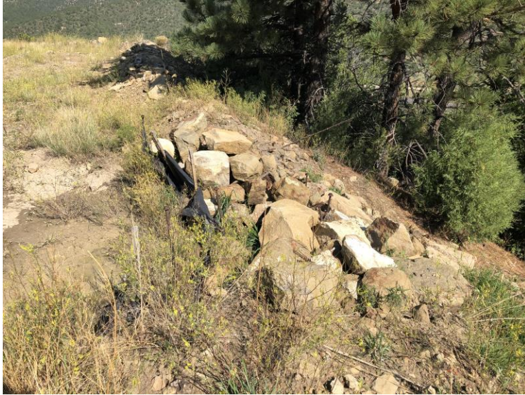
Riprap at runoff point for water tank pad
