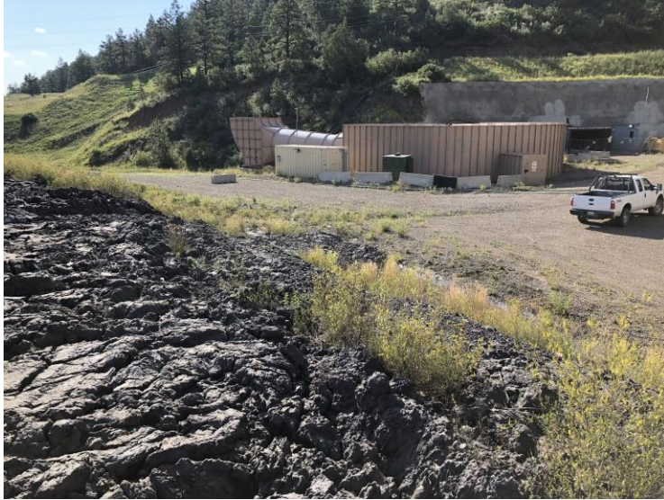
Pond cleaning material seeping off of clean coal storage area
