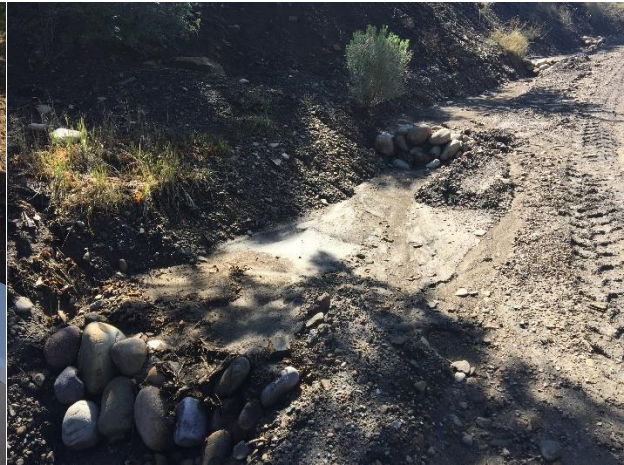
Photo 6 – Check Dams in Ditch ID-3
