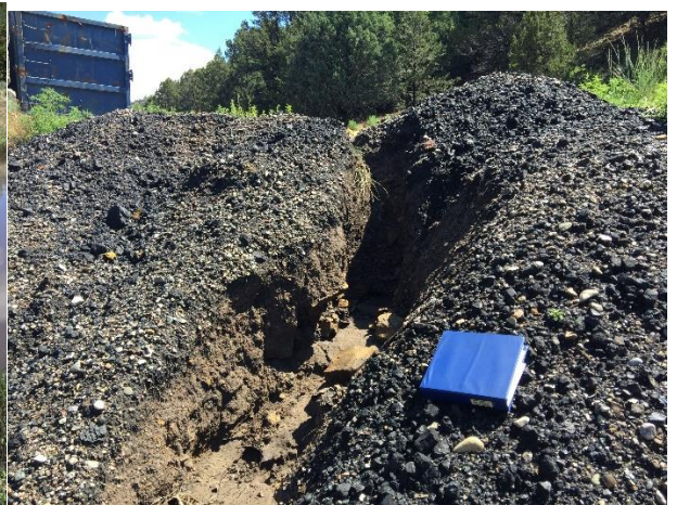
Photo 8 – Gully on NE Corner of Sediment Pond
