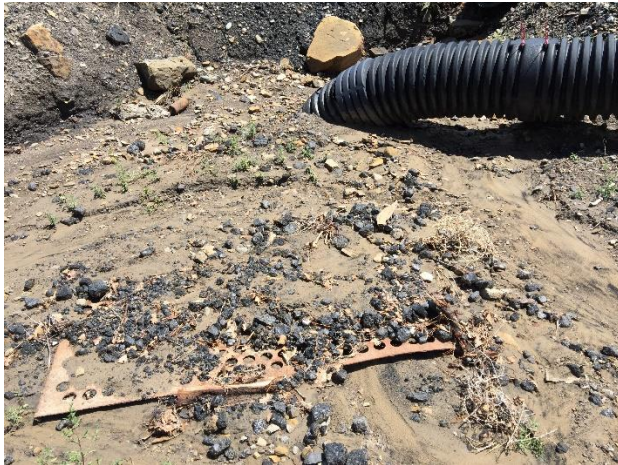
Photo 3 – Reach 7 Inlet Needs Cleaning
