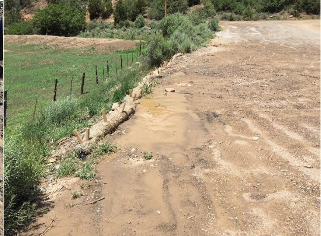
Photo 4 – Berm Needs to be Re-Built
