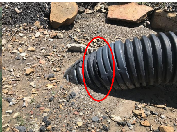
Photo 2 – Pipe Separation on Reach 3
