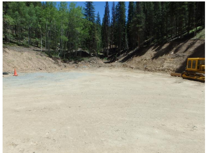
Pad area constructed with buried topsoil/reclamation material
