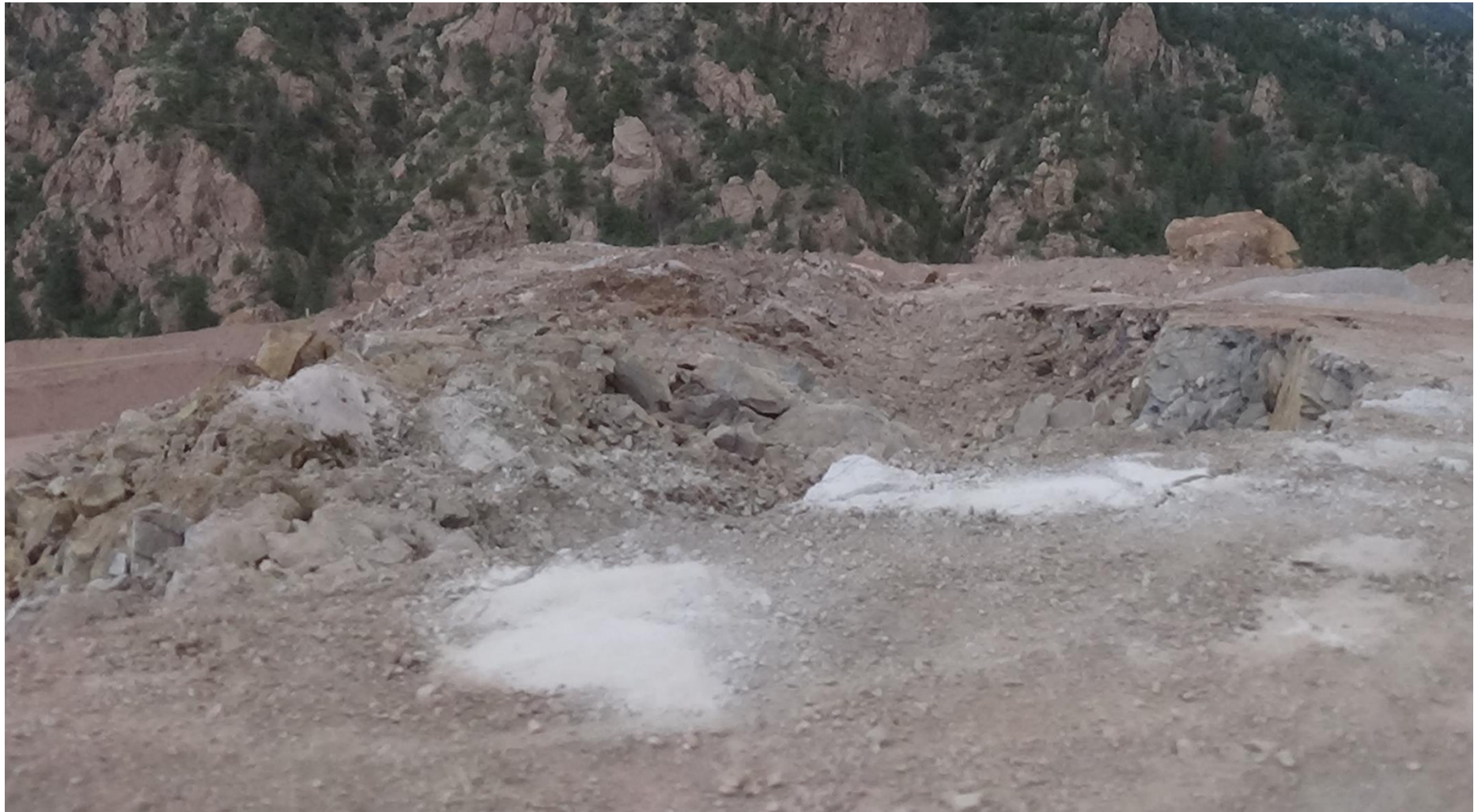
Post Blast And Backbreak
