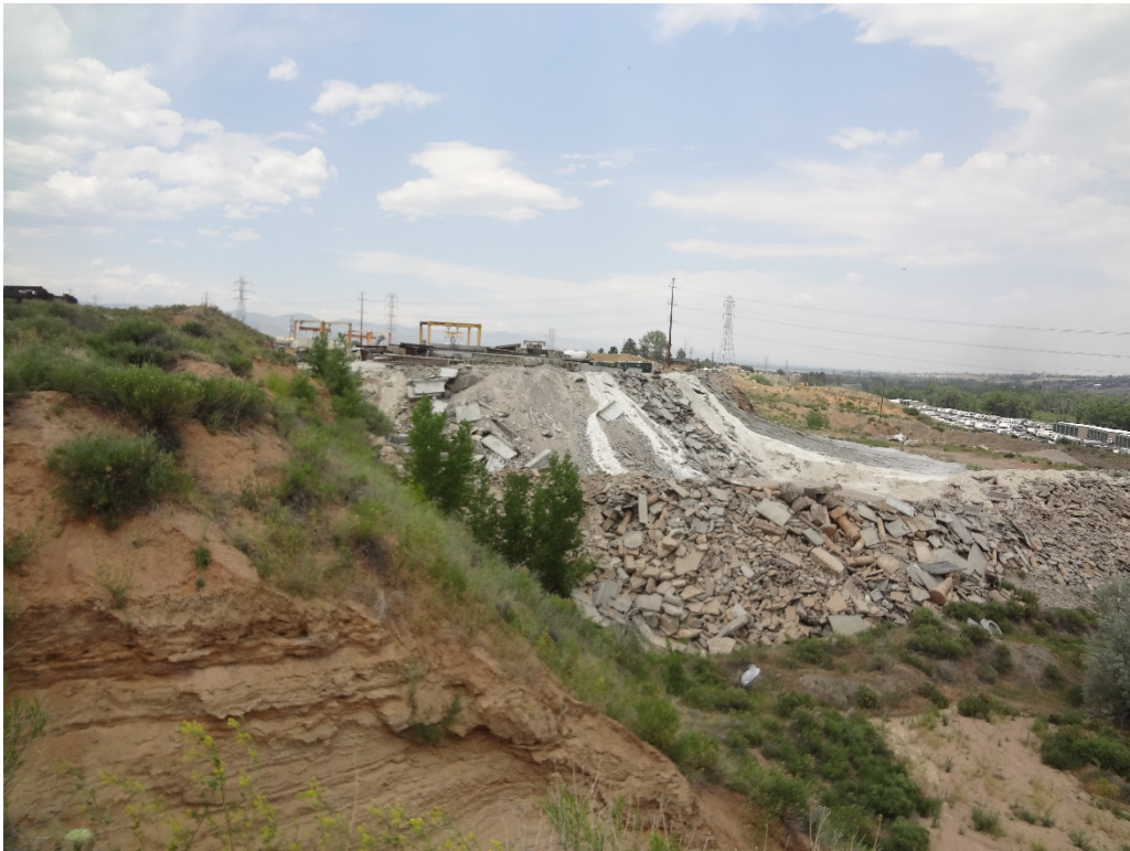
View of the site from the south highwall looking northwest
