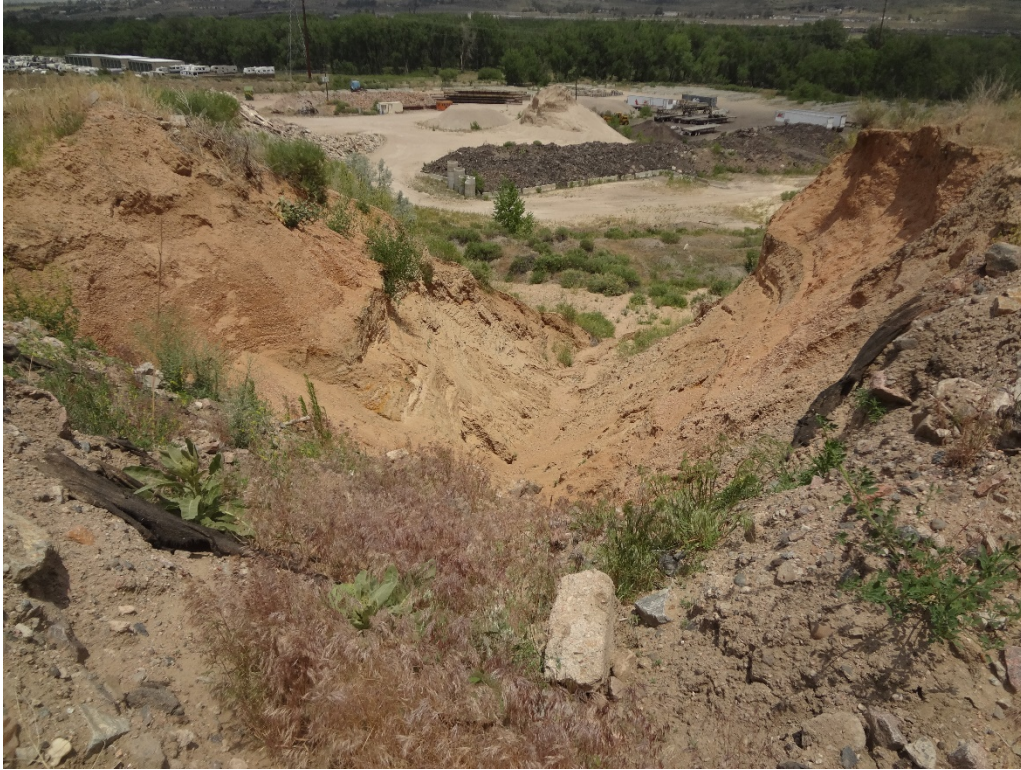
View of the erosion gully in the south highwall
