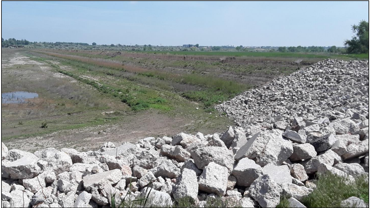
Photo 17. View looking northeast across eastern slope of East Reservoir, showing slope at 3H:1V gradient and stable with vegetative cover. This slope will be covered with rip rap, per City of Loveland, as was done with southern slope (shown in foreground).
