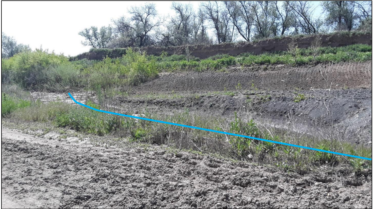
Photo 11. View looking south at southern edge of West Reservoir pit, with location of dewatering trench indicated by blue line. Tree-lined berm in background separates this pit from an unlined pond in the Kauffman Pit permit area. Water from the dewatering trench is pumped to the Kauffman Pit pond.
