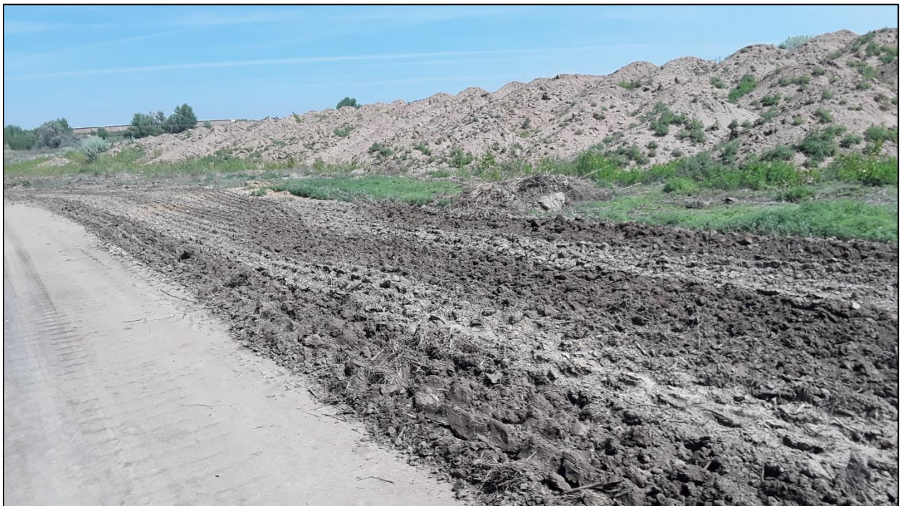
Photo 6. View looking north, showing topsoil stockpiles stored along eastern slope of West Reservoir.
