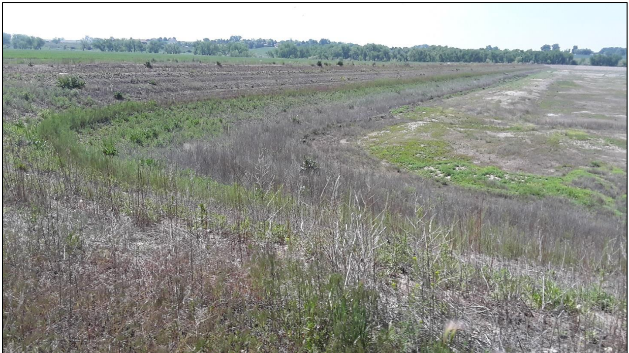
Photo 14. View looking southeast across eastern slope of East Reservoir, showing slope at 3H:1V gradient and stable with vegetative cover. This slope will be covered with rip rap, per City of Loveland.
