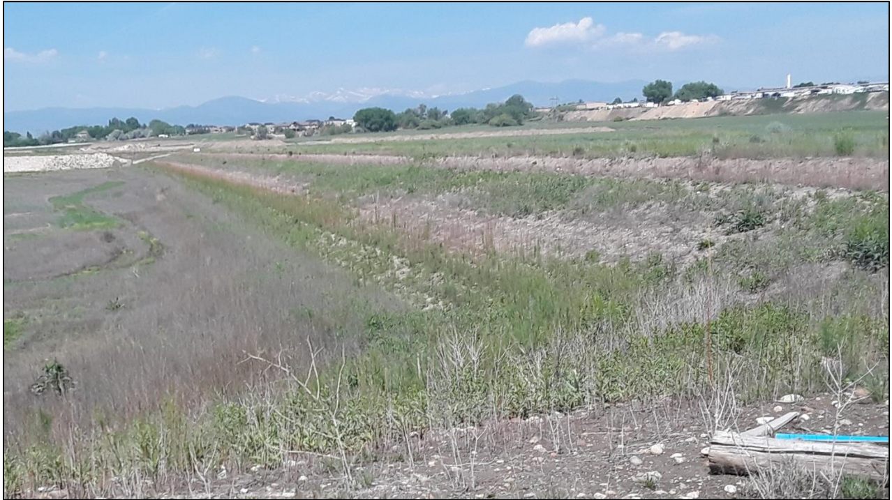
Photo 15. View looking northwest across northern slope of East Reservoir, showing slope at 3H:1V gradient and stable with vegetative cover. This slope will be covered with rip rap, per City of Loveland.
