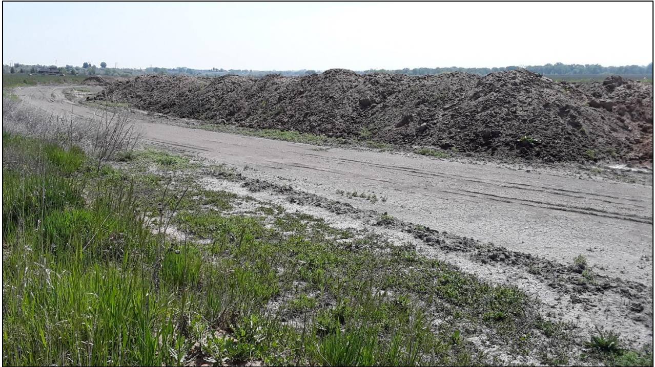
Photo 3. View looking south from outside of triangular area, showing topsoil stockpiled along northern edge of pit.
