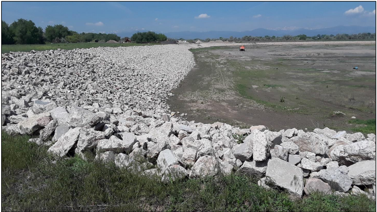
Photo 16. View looking west across southern slope of East Reservoir, showing slope at 3H:1V gradient and covered with rip rap composed of crushed concrete.
