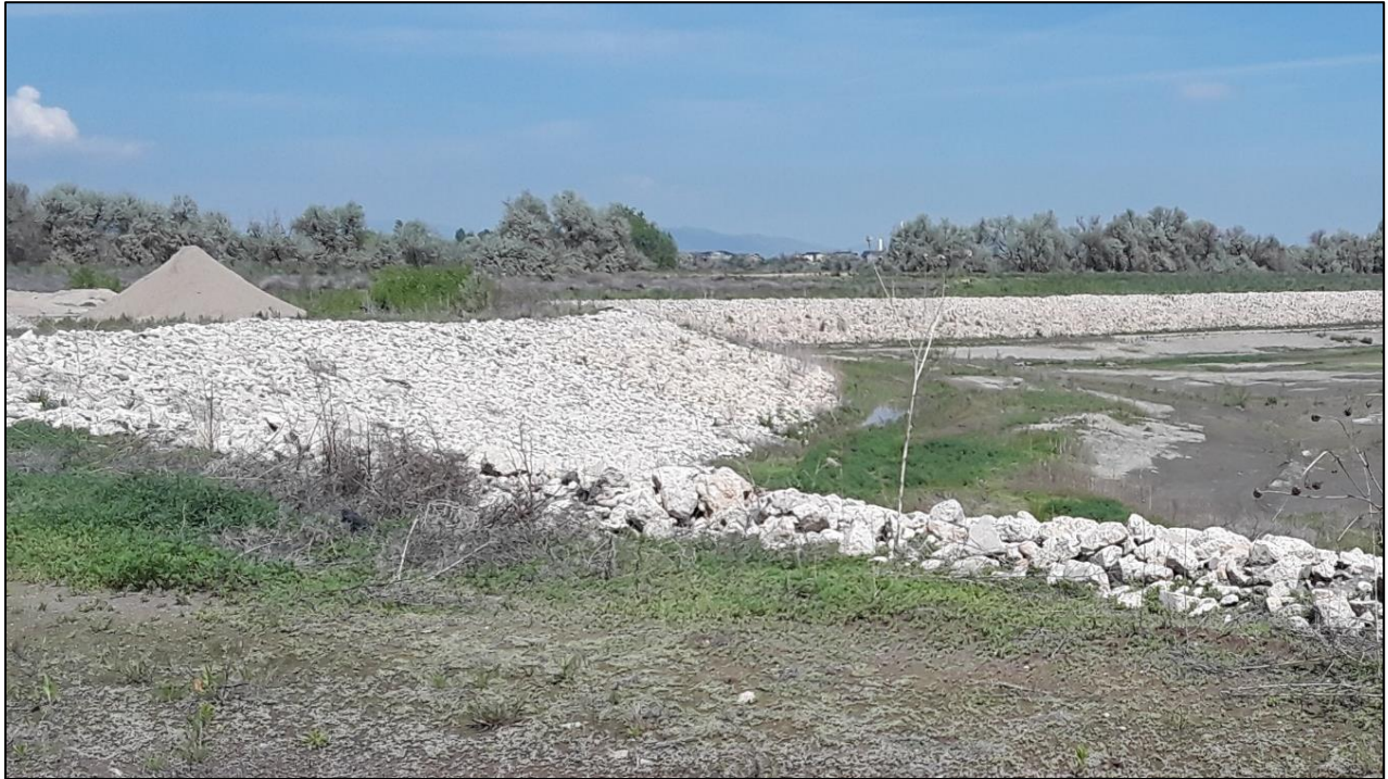
Photo 19. View looking northwest across southwest corner and south slope of East Reservoir, showing slope at 3H:1V gradient and covered with rip rap composed of crushed concrete. Stockpiles visible at left are part of Kauffman pit permit area.
