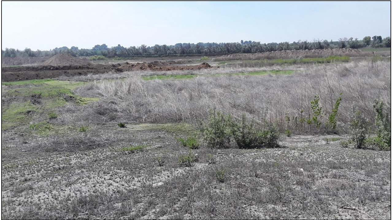
Photo 7. View looking south across floor of West Reservoir, from its northern edge.
