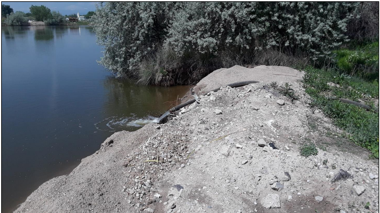
Photo 12. View from top of berm separating West Reservoir from unlined pond in Kauffman Pit permit area, showing hose discharging water to pond from dewatering trench in West Reservoir.
