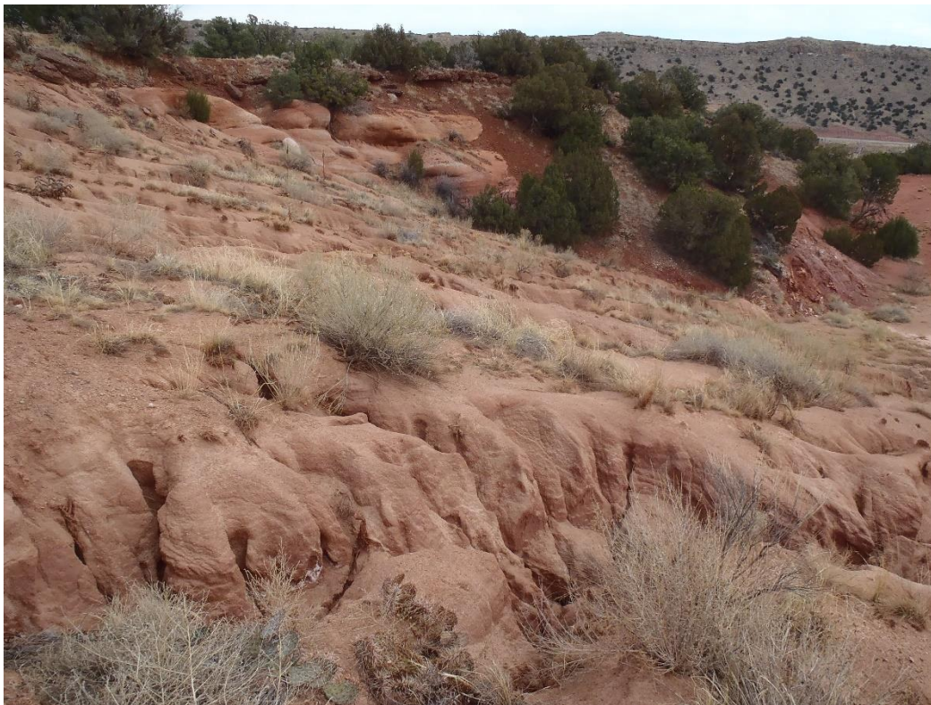
Photo 6. Highly eroded lower fines disposal area (looking NE).
