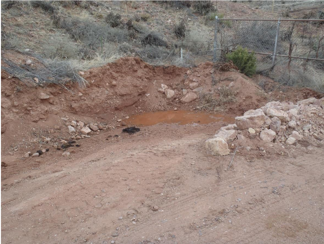
Photo 10. Sediment trap along access road (near entrance, looking east).
