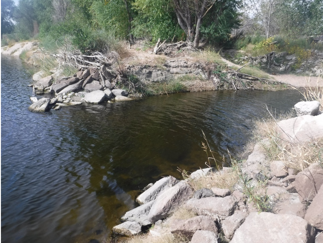
Cut outlet on the north side of Lake Robert in need of stabilization and armoring; looking northwest.
