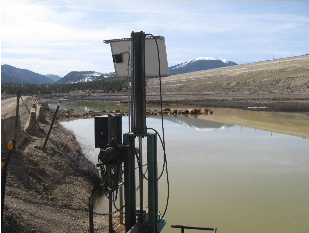
5. Seep Water Collection - seep water gate connecting main canal to diversion ditch.
