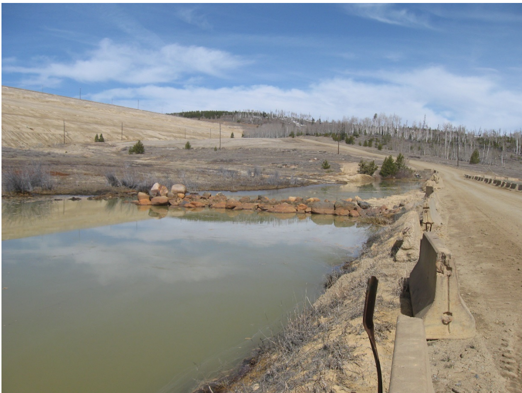
4. Seep Water Collection - main collection canal.
