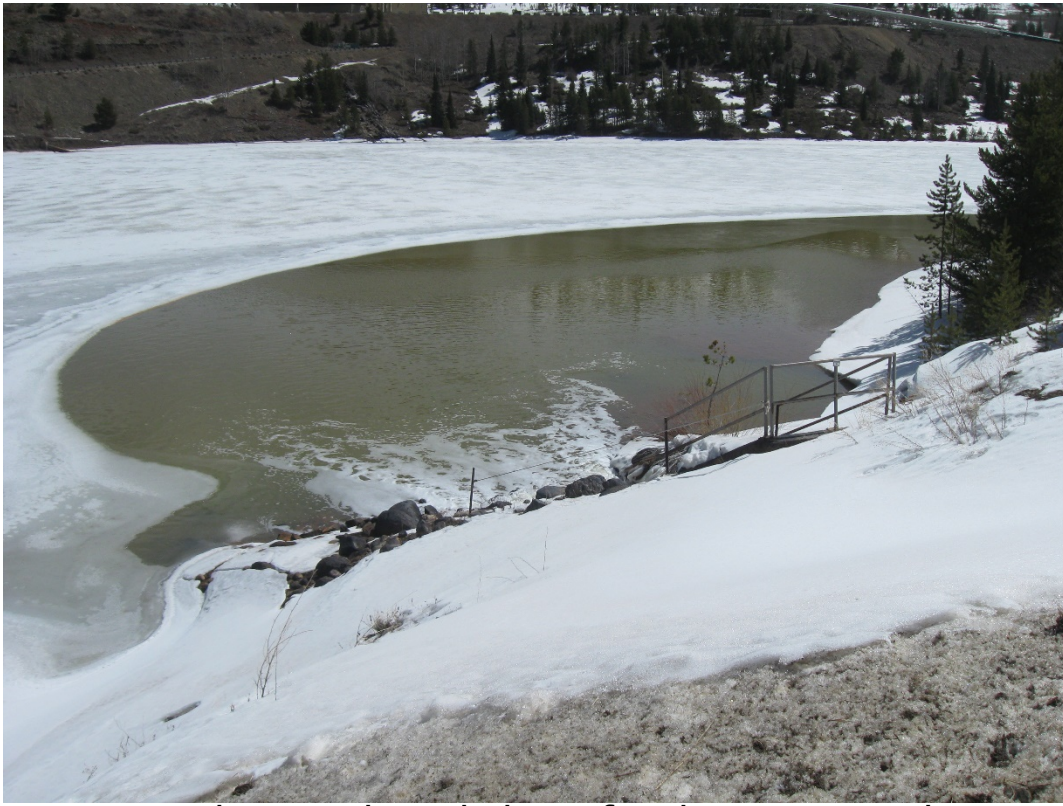
1. East Branch Reservoir - Discharge from barge pump station.
