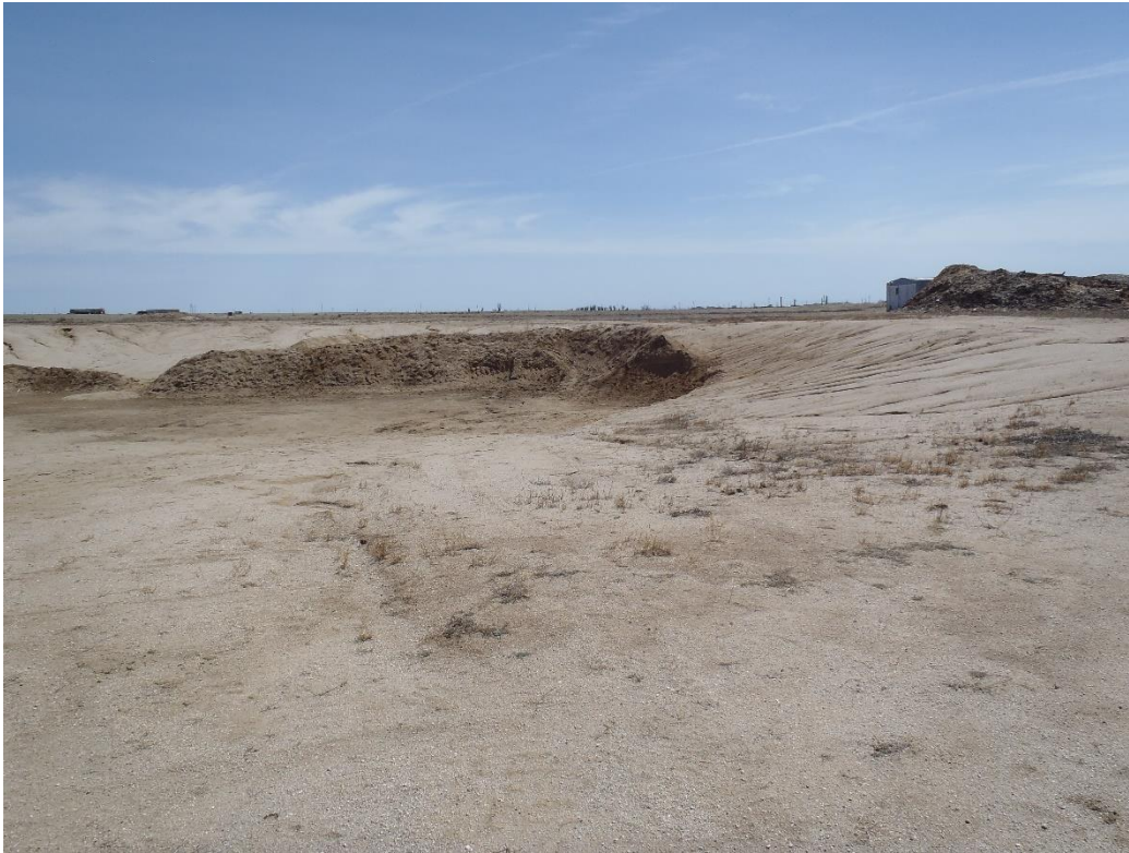
Photo 2. North (left) and west (right) highwalls sloped at 3H:1V or flatter.
