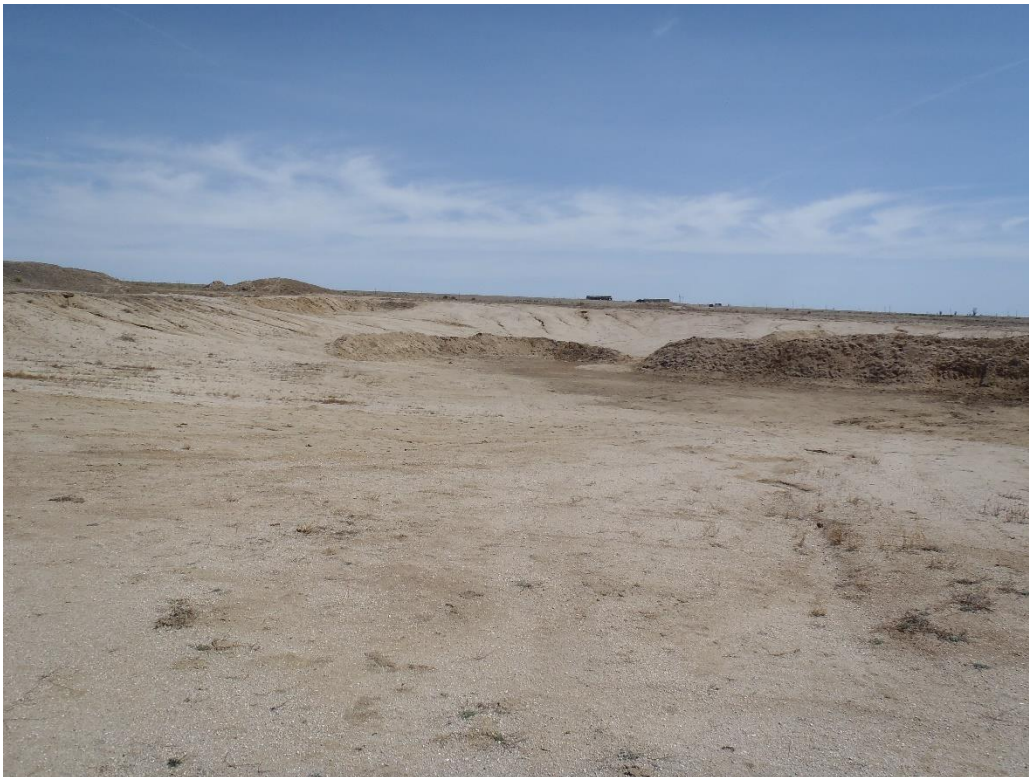
Photo 1. East (center background) and west (foreground) highwalls sloped at 5H:1V or flatter (looking NE).
