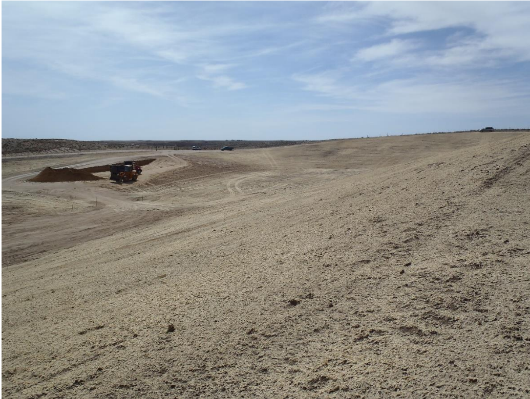
Photo 4. Hydromulched west and south slopes (looking SE).
