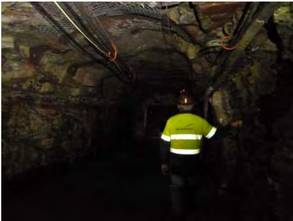
Figure 15 - Existing Rock Bolts, Chainlink Mesh, and Mine Strap Support (Outby of Air Door)
