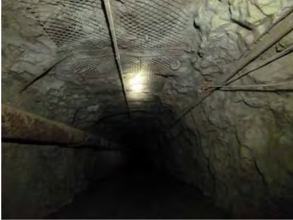
Figure 16 - Existing Rock Bolts, Chainlink Mesh, Mine Strap, and Flashcrete Support
