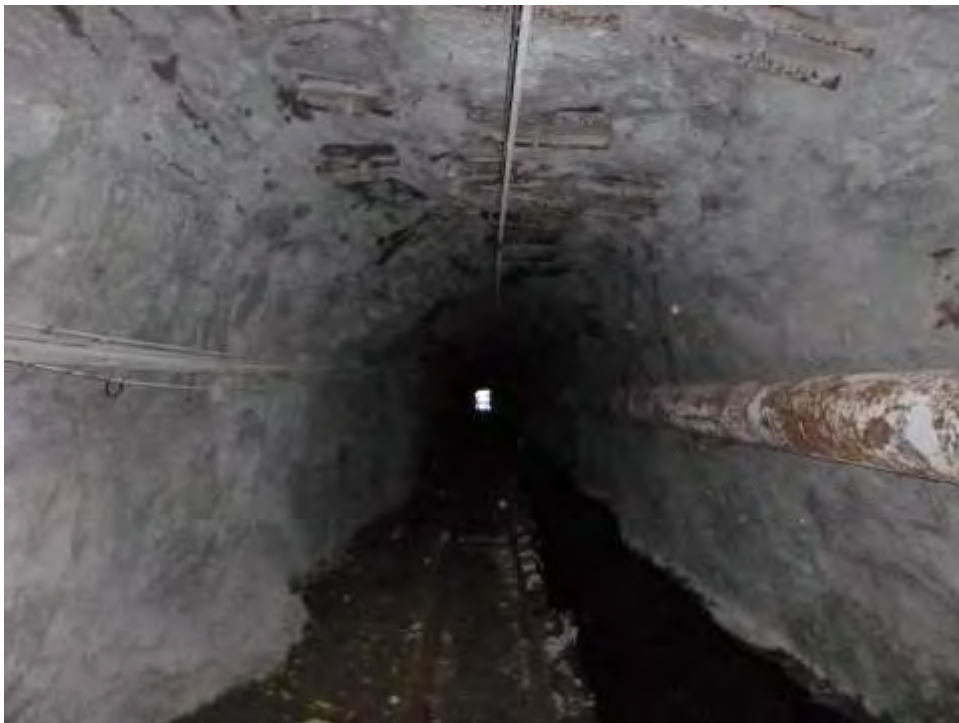
Figure 17 - Existing Rock Bolts, Channel Plates, and Flashcrete Support
