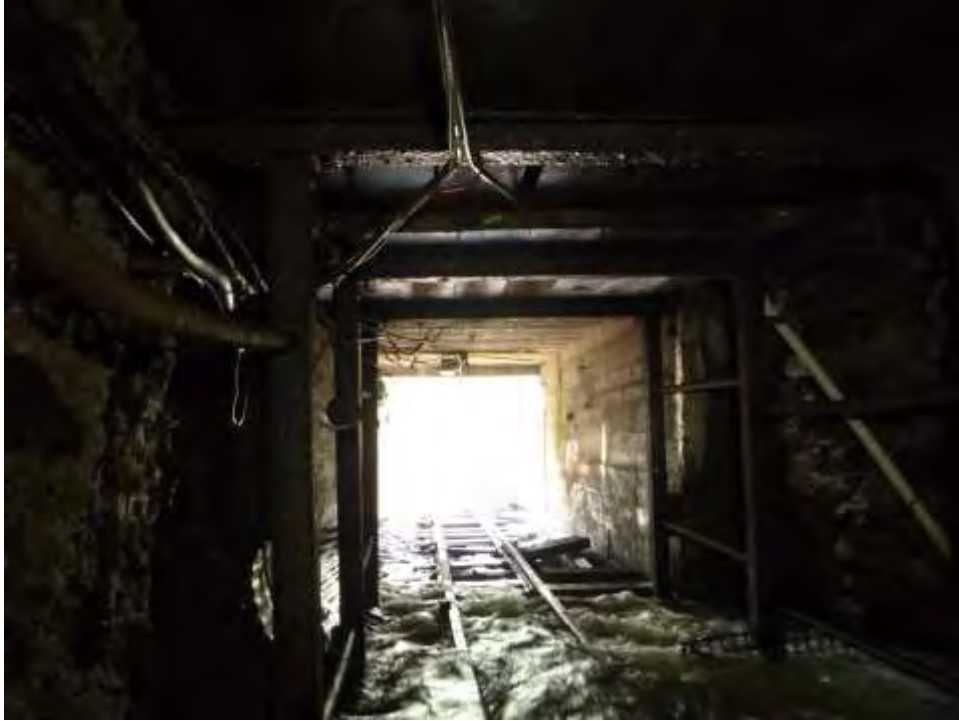
Figure 14 - Existing Steel Sets and Concrete Box Structure (looking out of portal)
