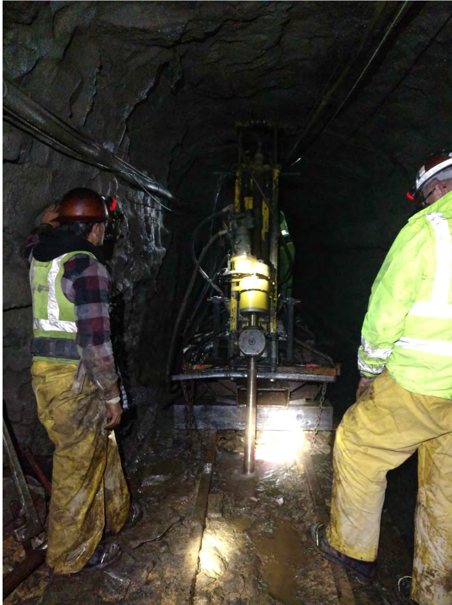
Figure 6: Drilling Operations for Exploratory Borehole D-1
