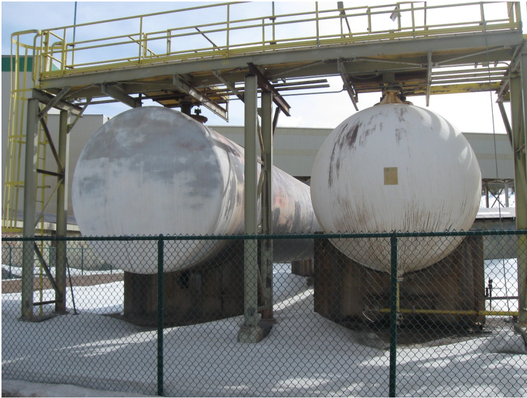
3. Hydrochloric Acid Storage Area.
